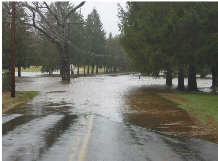
A flooded roadway in Connecticut (CT DEP).
