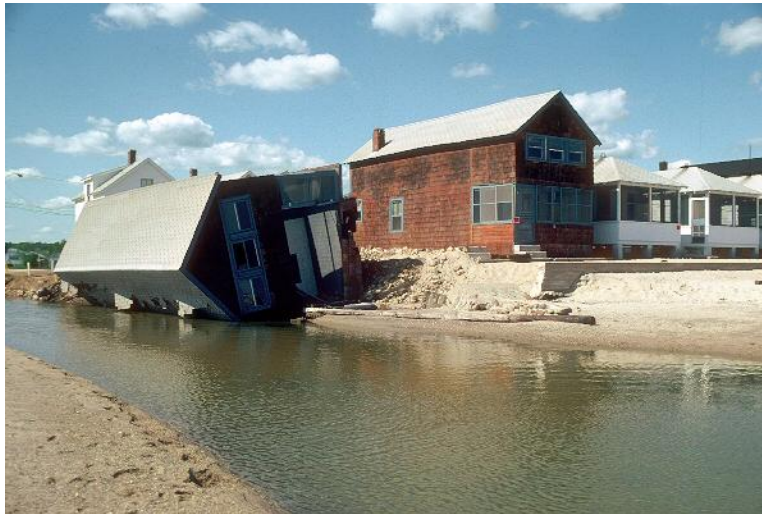
Undermining and collapse of a house caused by coastal flooding that was intensified by an undersized culvert (CT DEP).
