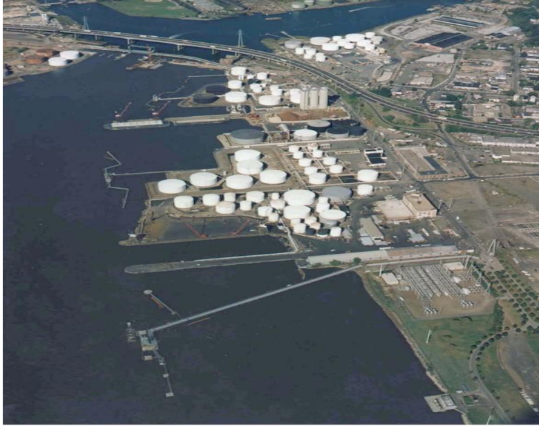
Coastal fuel tanks at the port of New Haven (CT DOT).
