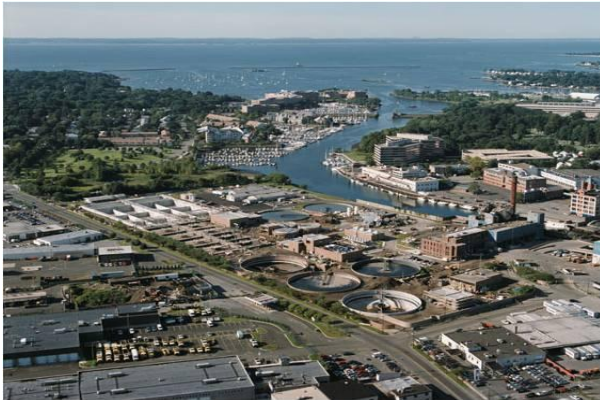
Wastewater treatment plants located near Long Island Sound, like this one in Stamford, may be at risk from sea level rise (CT DEP).
