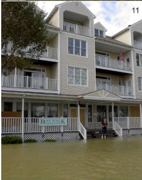
Photos 9–15. Chesapeake Beach and North Beach the Day after Isabel. The beach at Chesapeake Beach has almost all been replaced by stone revetment, which protects against erosion but not high water (9). The new condominiums have first floors elevated to the base flood elevation, but owners suffered substantial uninsured losses because most had improved the floor below the first floor. As late as 2:00 p.m., the Bay was still over the road between Chesapeake Beach and North Beach (10), and several feet deep throughout low-lying areas of North Beach (11–12). The most severe damage occurred along the boardwalk section of Atlantic Avenue (13), although flooding was also severe along the avenue's paved portion (14–15).
