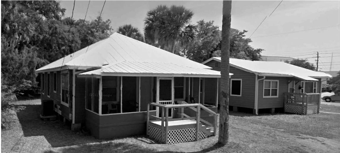
Fig. 35: Vernacular frame houses in the Lincolnville district were originally constructed on block piers, some coquina. The added height currently protects from repetitive flooding in the area. This area on Duero Street, the district's western border, is likely to be flooded by 2100. [Google Earth; street view photograph, 2013]
