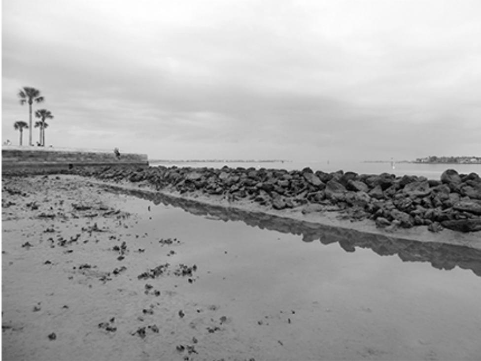
Fig. 41: The rip-rap seawall, as seen at low tide, was constructed by the NPS to reduce erosion on the historic seawall and to create a natural habitat. [Ann Horowitz; photograph, January 2013]
