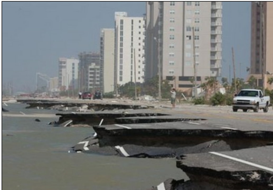
Figure 2.5. Storm surge damage to State Road 128 in Orange Beach, Alabama from Hurricane Ivan in 2004 (Source: Hurricane Ivan, 2004).
