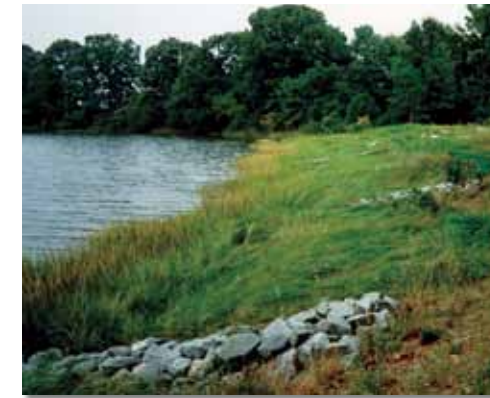
Sea-level rise contributes to the erosion of approximately 580 acres of shoreline per year. Maryland's Living Shoreline Protection Act of 2008 requires that living shoreline or non-structural shore protection practices be used wherever technologically and ecologically appropriate. Living shorelines provide erosion control benefits while also enhancing the natural shoreline habitat. They often allow for natural coastal processes to remain through the strategic placement of plants, stone, sand fill, and other structural and organic materials.
