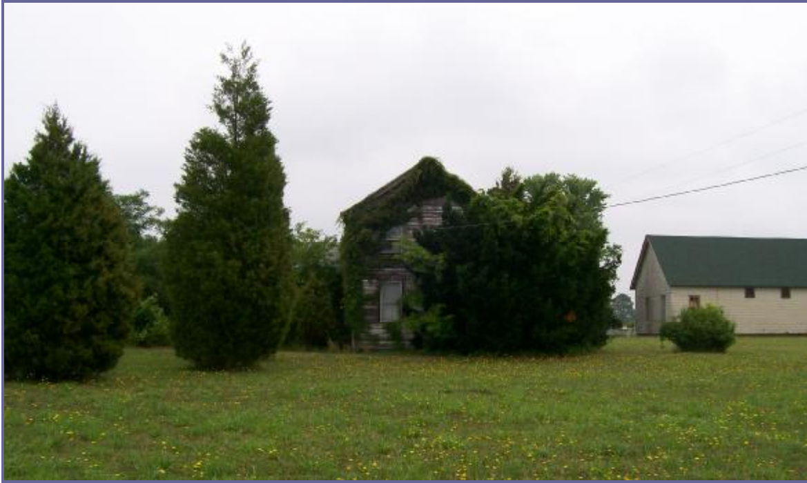
Abandoned property on Elliott Island Road.
