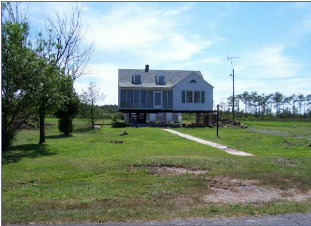
A Toddville Road home damaged by Tropical Storm Isabel in 2003 is elevated using FEMA funds in 2006. From the road, appearances are deceiving; behind and across the street from the house are extensive areas of high marsh and tidal channels.
