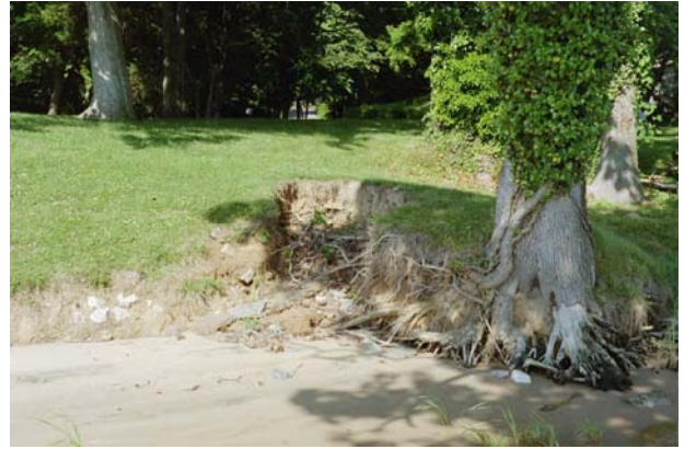
Figure . Epping Forest, Section 2, bank erosion
