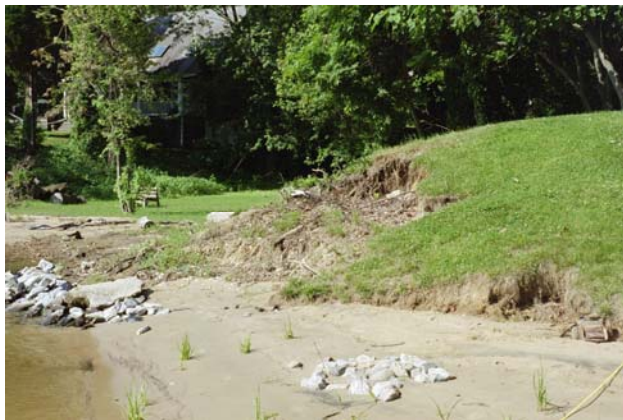
Figure . Epping Forest, Section 1, bank erosion
