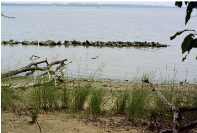
Figure . South River, Station 1+32, water
