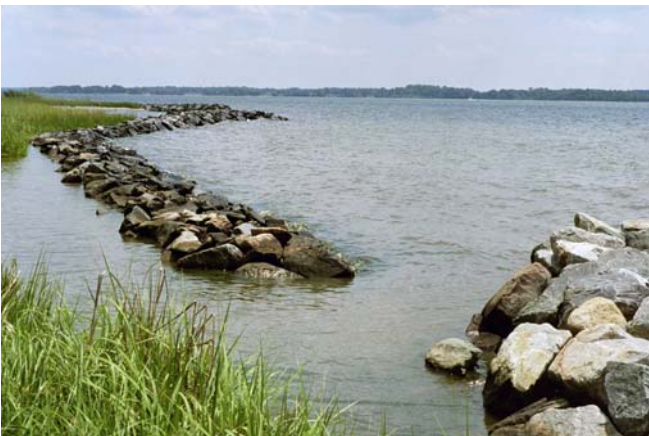
Figure . JP Park, Station 28+11, sill window
