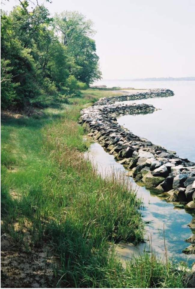
Figure . JP Park, Station 28+11
