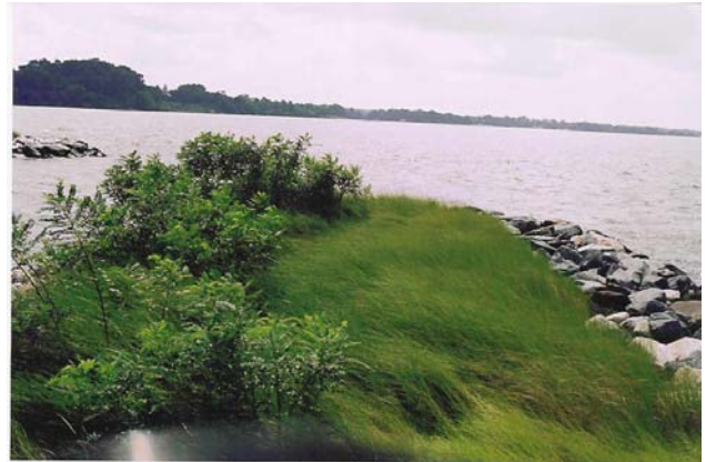
Figure . JP Park, Station 48+60, planter breakwater
