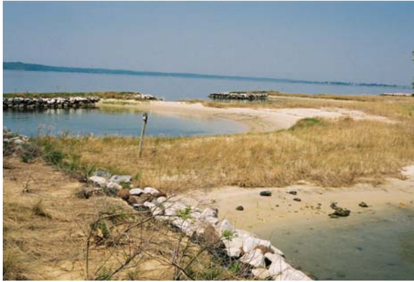
Figure . JP Park, Station 48+60, left
