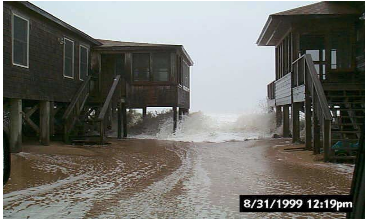
Figure 8: Storm Overwash from Tropical Storm Dennis Between Two Buildings in Kill Devil Hills, NC
