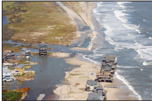
Storm surge from Hurricane Irene washes out NC 12 on NC's Outer Banks. Just North of Rodanthe. 08/2011
