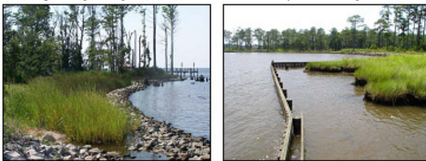
Figure 3.12 View of a rubble mound sill (left) and a timber sheet pile sill (right) (Bendell et al., 2006).
