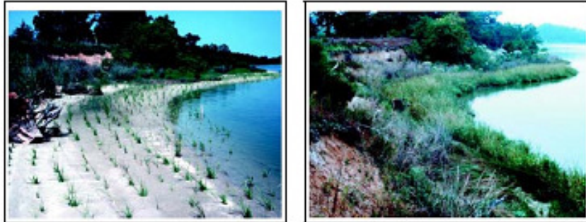
Figure 3.11 Marsh planting as vegetation control (left) and one year later (right) (Bendell et al., 2006).
