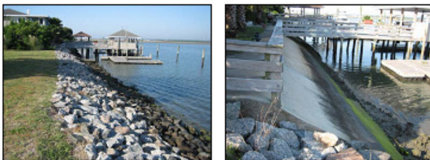
Figure 3.13 Sloped structures constructed from rock (left) and watertight cast concrete (right) (Bendell et al., 2006).
