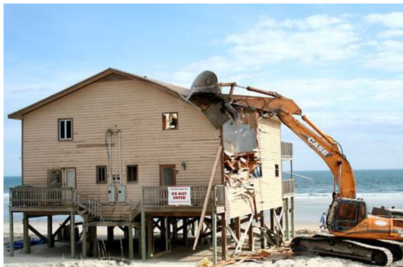
Figure 2.1 Four years after being condemned, the town of North Topsail removes structures from the beach. Photo Source: Connie Pletl, http://carolinacoastonline.com/articles/2009/03/04/topsail_voice/news/doc49ae92cf94719645792078.ppt
