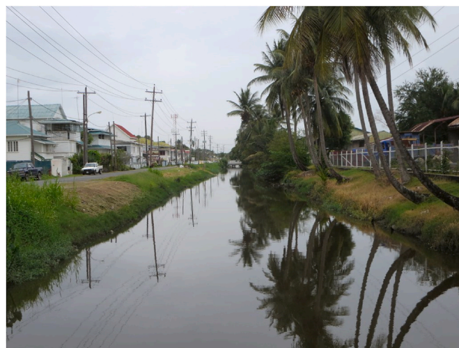
Fig. 5. Drainage canal along Cowan Street in Georgetown. (Source: David Stanley/Flickr under Creative Commons License 2.0)
