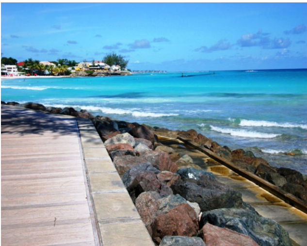
Plate 1. Protective measures used along the southwest coast of Barbados to minimise beach erosion. Source: Author's elaboration.
