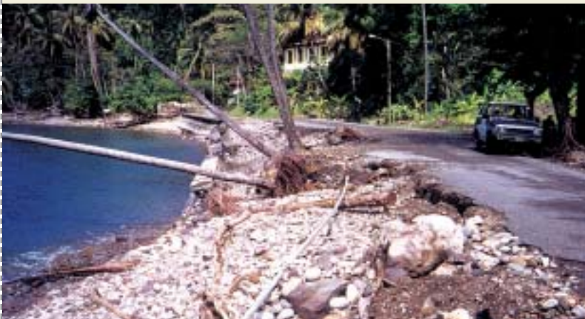
In 2000, after three major hurricanes, Toucarie Bay was a narrow strip of stones and the coastal highway was seriously damaged
