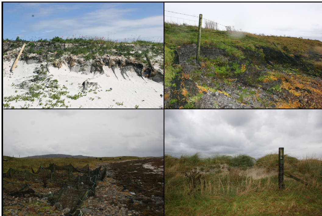
Fig. 6. Photos of the ridge at Kilpheder showing clockwise from top right: eroded scarps on the sea-ward side of bund (March, 2012); the top of the ridge, partly re-vegetated following over-topping during winter 2012–2013 (March, 2013); damaged sand traps made from fishing nets, located to the south of the ridge (March, 2012); sand accumulation in the eroded scarps at the base of the seaward side of the bund (June, 2012).
