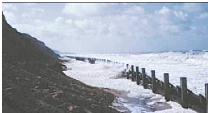
Pressure on coastal defences from rising sea level is already increasing. © M Robinson.
