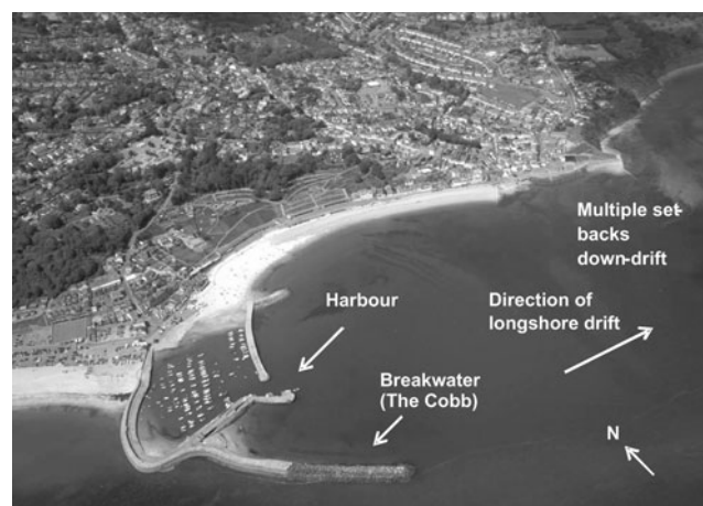
Fig. 8 Progressive multiple set-backs down-drift of Lyme Regis, Dorset. 2007 aerial photograph. Photograph courtesy of West Dorset District Council
