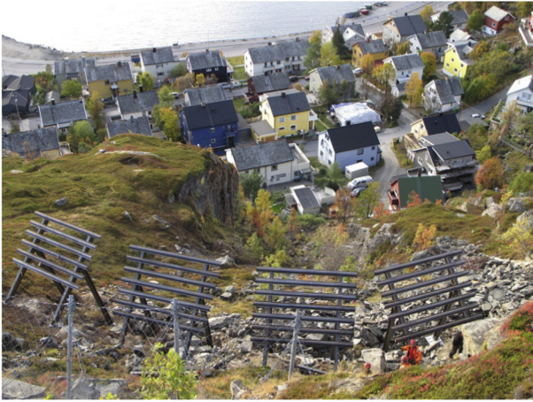
Fig. 3. Example of avalanche protection measure in Hammerfest.
