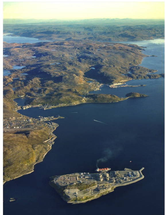
Fig. 2. The LNG plant is located on a small island (Melkøya), close to Hammerfest.
