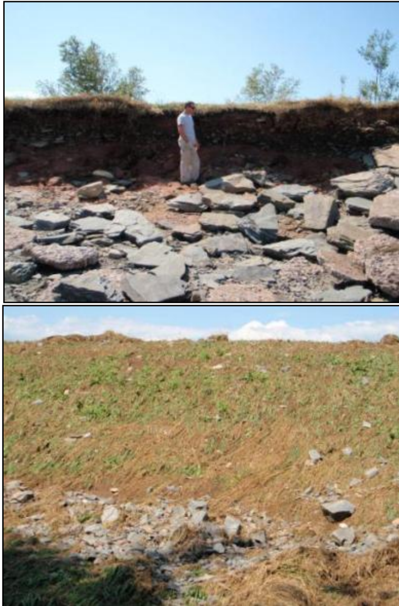
Figure 3: Impacts of Hurricane Bill on dyke at Noel (NS24) in August 2009. a) erosion and undercutting of earthen dyke structure and removal of shoreline armouring, b) armouring rocks transported to the landward side of the dyke by wave action and overtopping.
