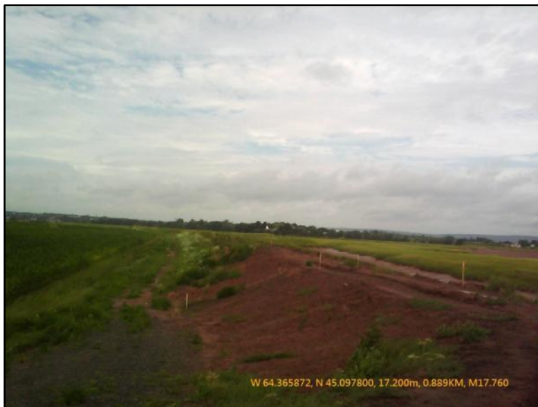
Figure 59: Surficial erosion of dyke surface at NS65 next to Wolfville Waterfront Park. Photo taken July 5, 2011.
