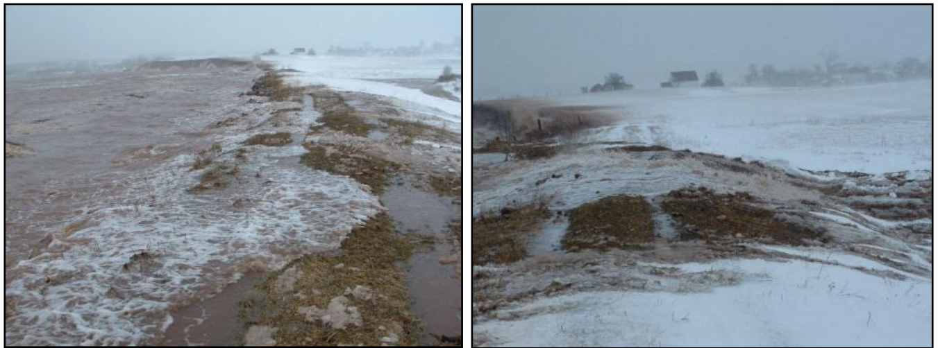
Figure 25: Storm impacts on Feb 1, 2006 at the Avonport Dyke. a) storm waves battering marsh; b) storm surge reached upper limits of dyke and dyke overtopped. Photo by T. Hamilton, 2006.
