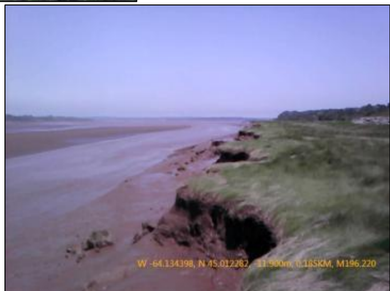
Figure 68: Eroding foreshore along Newport marsh, Avon river. Photo taken July 5, 2011.
