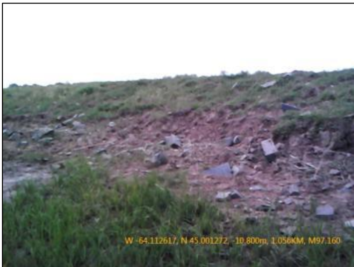
Figure 67: Dyke toe scour and erosion of armouring at Station 'Q' Figure 64 Photo taken July 4, 2011.
