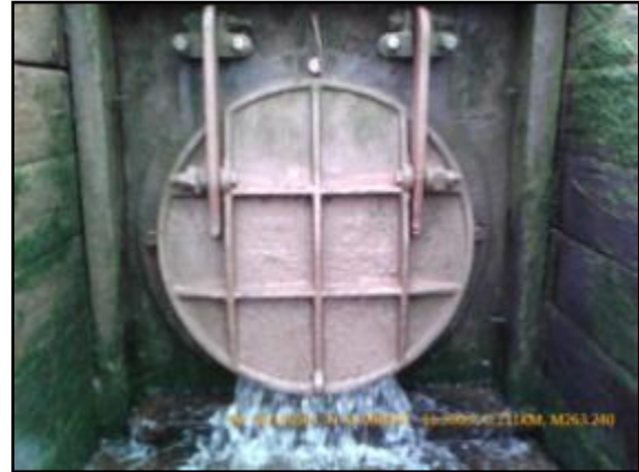
Figure 4: Modern aboiteau structure Grand Pre Marsh Summer, 2011
