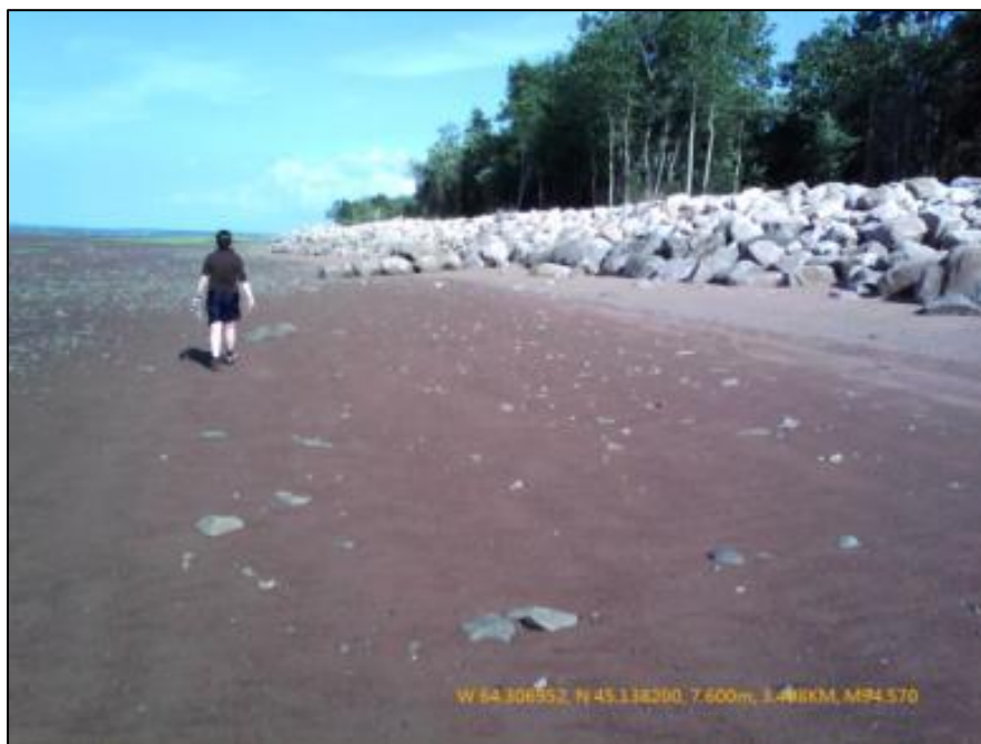
Figure 53: Rock armoring along the backshore near Evangeline beach likely placed by property owners indicated by 'J' on Figure 50. Photo taken July 21, 2010 (Pietersma-Perrott and van Proosdij, 2012).
