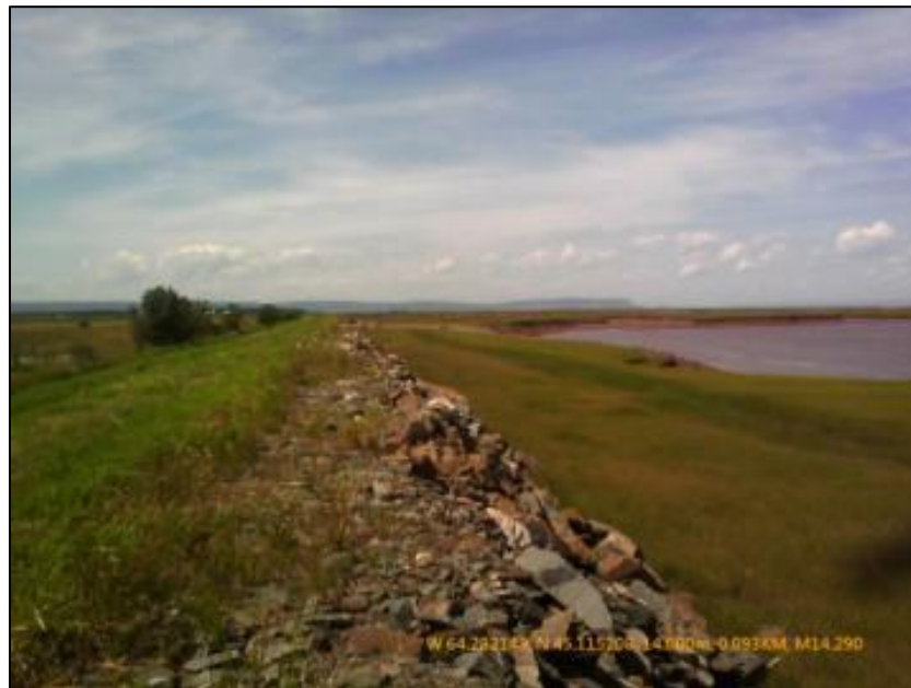
Figure 49: Eroding foreshore marsh and armoring along the backshore along the Gaspereau R. Indicated by 'H' on Figure 48 Photo taken July 23, 2010. (Pietersma-Perrott and van Proosdij, 2012).
