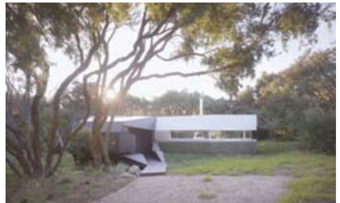
The Cape Schanck House by Paul Morgan Architects has been sensitively sited and designed to respond to the surrounding coastal tea tree.
