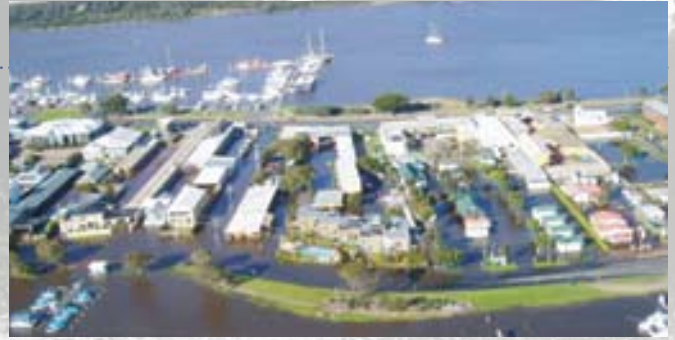
The flooded streets of Lakes Entrance during the floods of July 2007
