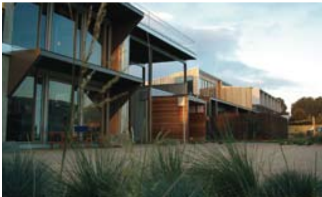
The Apollo Bay YHA by Perkins Architects incorporates numerous ESD principles and indigenous landscaping .
