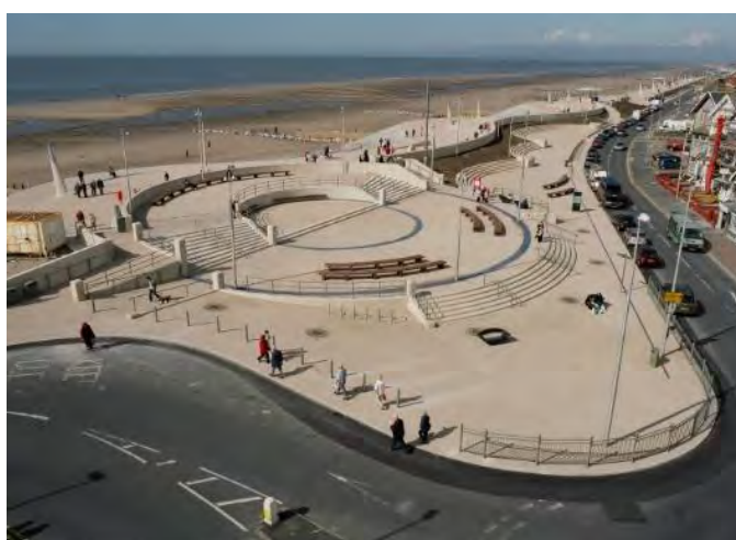
Figure 5-7 Coastal defence at Cleveleys, United Kingdom 5
