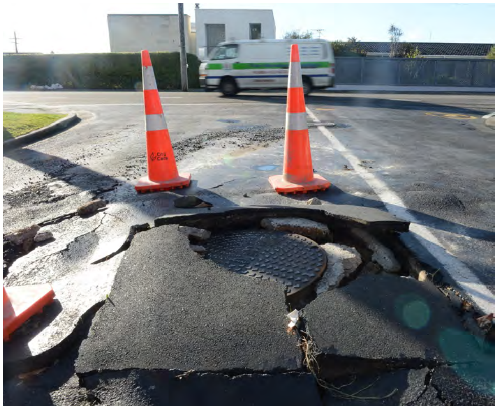
Figure 5.2 Heavy rainfall caused flooding and damage in Dunedin in June 2015 when the stormwater system could not cope with the deluge.
