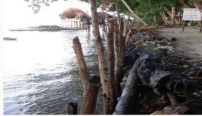
Figure 5. An example of a seawall built with local materials to prevent erosion (photo: Peter Bosip, July 2011)
