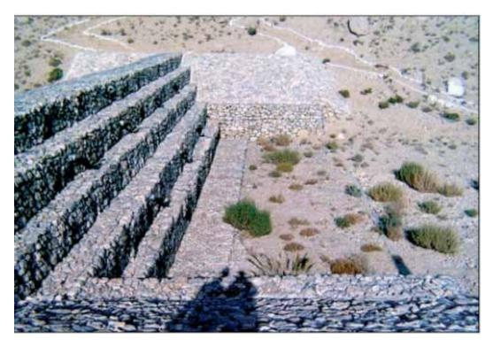
Leaky Check Dam in Balochistan for Groundwater Recharge.
