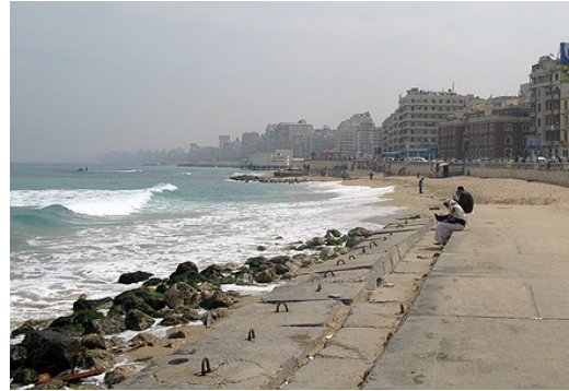
Fig 5 Rising water levels in the Mediterranean Sea are causing the barriers that line Alexandria, Egypt's Eastern Harbour, to slowly break down. (Hansen, 2008 )
