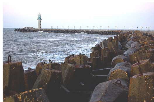
Fig 4 Sea barriers at Damietta, insufficient for combating the rising sea levels. (Russmerritt, 2008)
