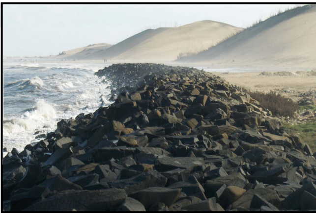
Figure 5: Shoreline at the middle delta coast: protection works and sand dunes. Source: El-Shinnawy [17].
