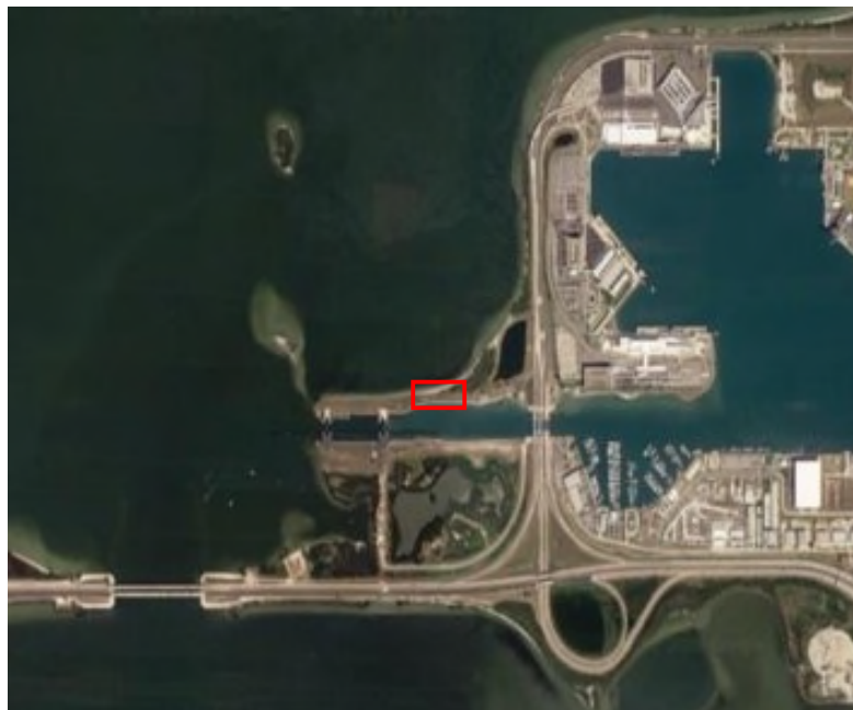
Figure 5-9: Canaveral Lock aerial view with proposed location for weir structure outlined in red (Google Earth 2019).
