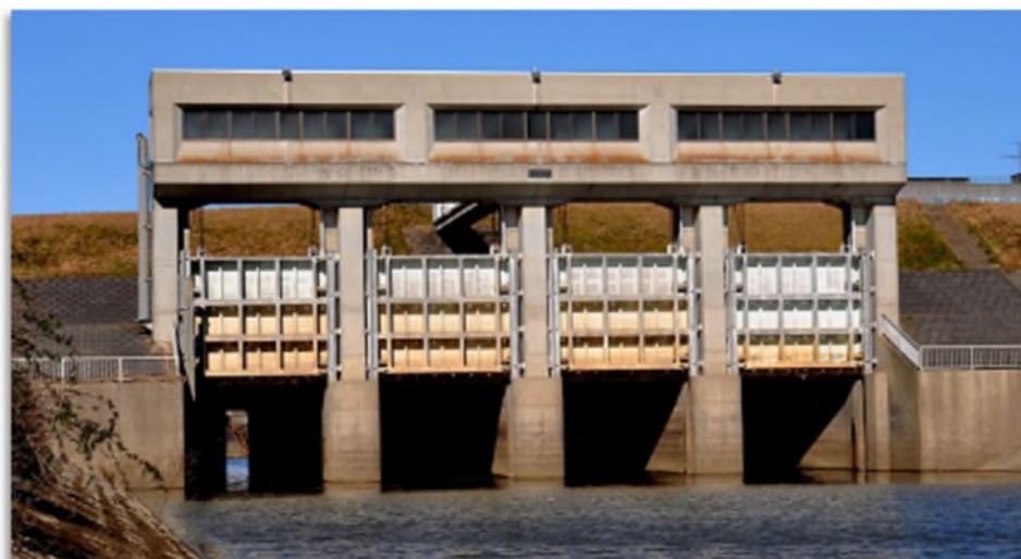
Figure 2-21: Example weir gate system (Pxfuel 2020)
