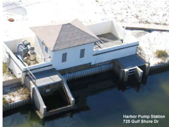
Figure 6. Destin Harbor Pump Project Pump Station (Indian River County 2016)
