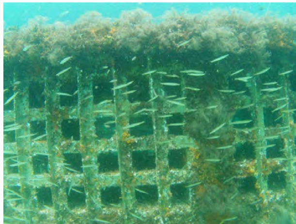
Figure 7. Destin Harbor Pump Project Gulf Intake (Indian River County 2016)
