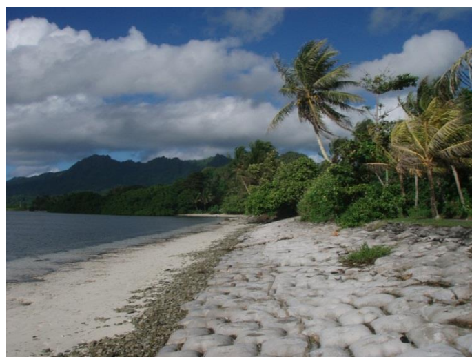
Seawall of cement bags in Lelu. Photo: Iris Monnereau
