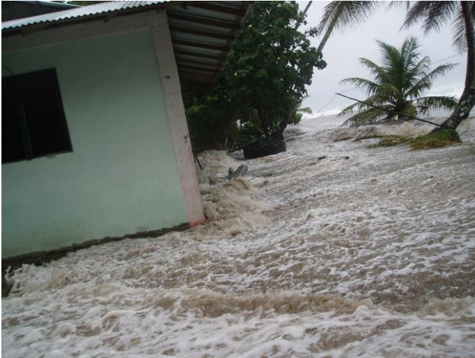
The house of Alokoa Jonithan (taken from a tilted position), during the 2008 extreme event (box 5.2 and 5.4). Photo: Carlos Cianchini
