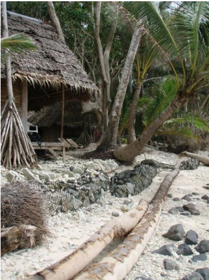
One of the cabins at Katrina's hotel by the beach and the gabion that she placed in front of it filled with rocks and dead coral (box 4.2 and 4.4). Photo: Carlos Cianchini
