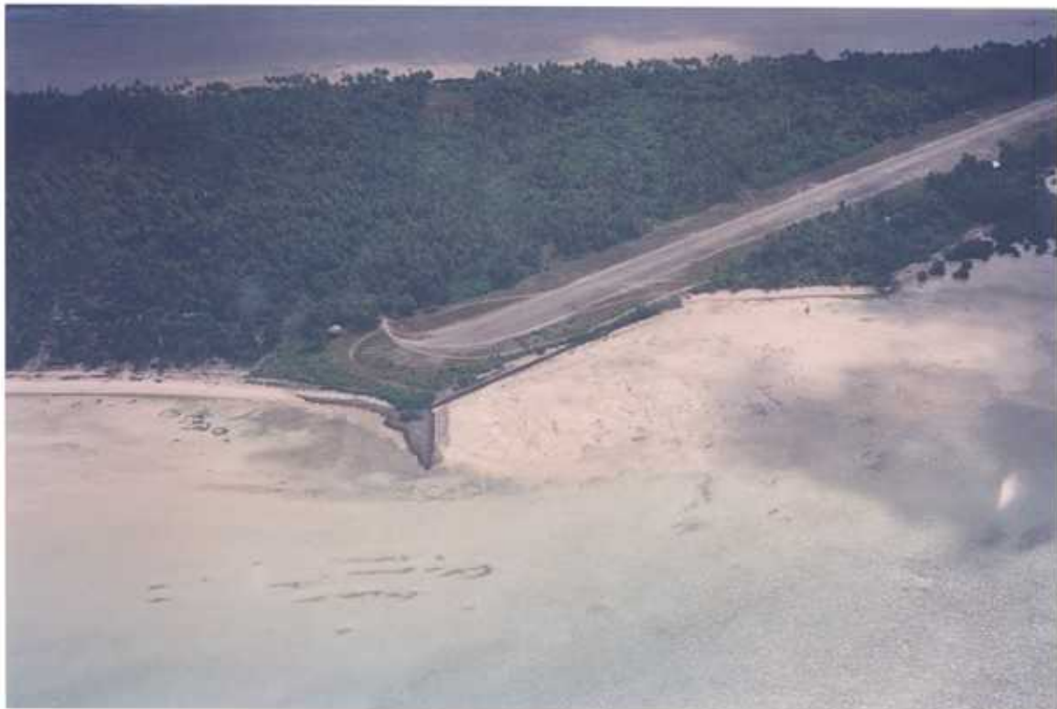
Figure 32. Rotima Island (Site 2: west end of airfield), Nonouti. View northeast of lagoon shoreline. Airfield shoreline reclamation with gabion basket seawall extends east (right) of conglomerate platform in centre of photo.
