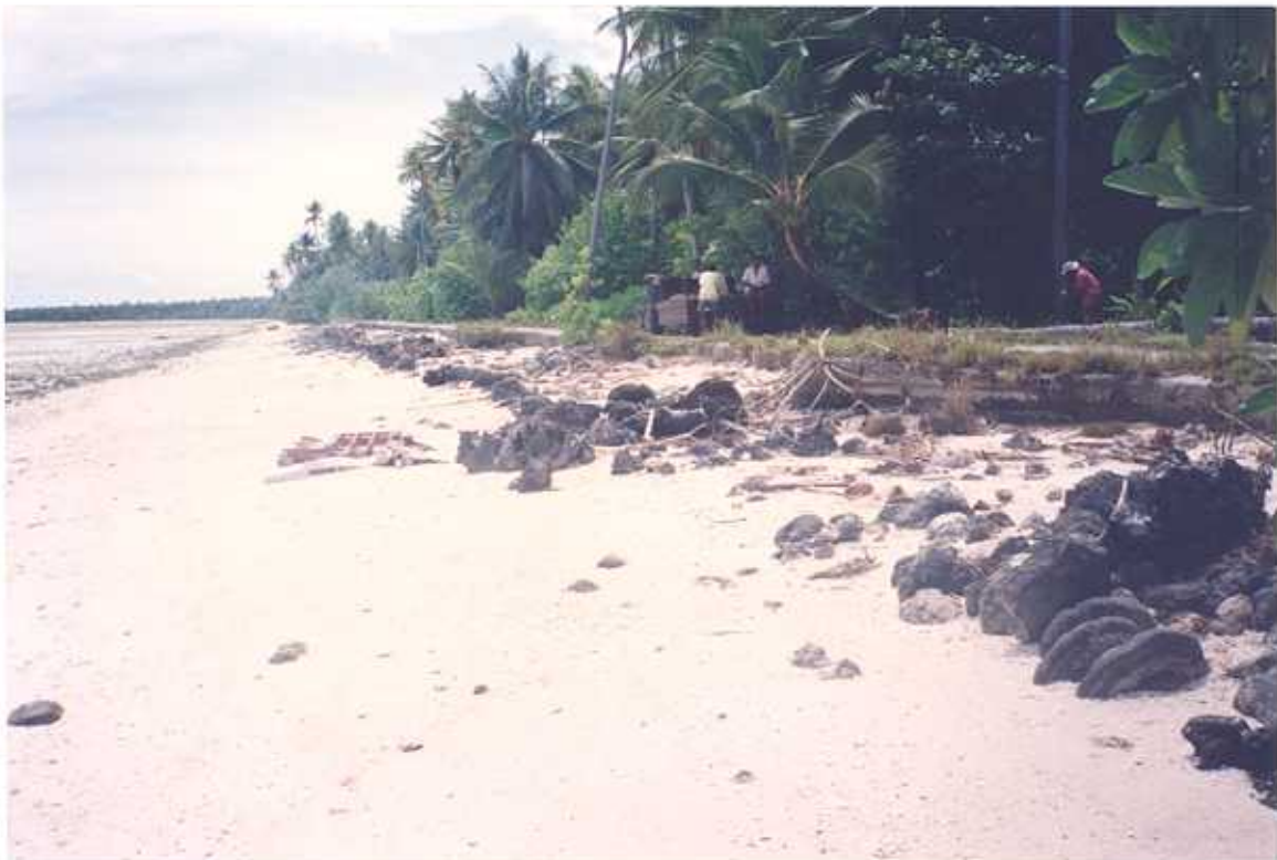
Figure 43. Tanimainiku (Beach Profile: 2), Abemama. View northwest past location of beach profile. Note severe erosion of road and remains of seawall constructed from coral rubble and boulders including whole micro-atolls.
