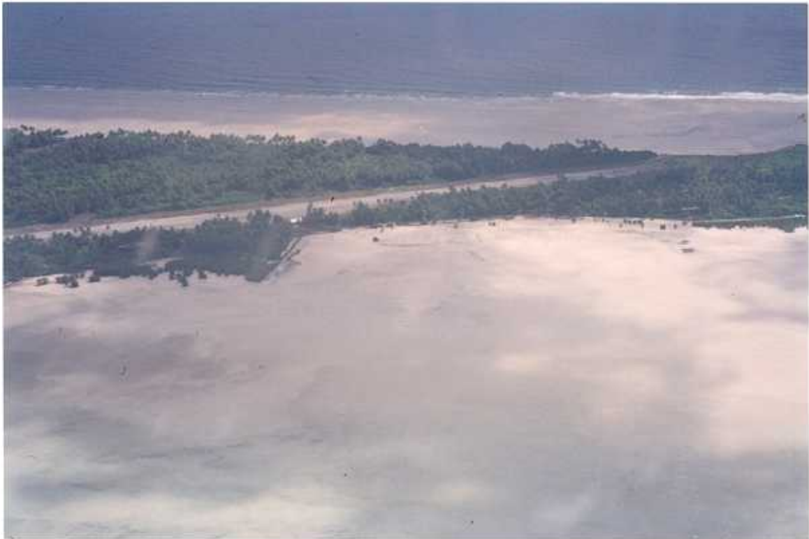
Figure 31. Rotima Island (Site 1: airfield road), Nonouti. Oblique aerial view northeast towards lagoon shoreline and airfield. Road along shoreline in middle of photo is being undermined by coastal erosion.
