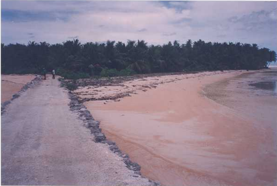
Figure 9. Nikutiri Island, Tabiteuea South. View south to Nikutiri Island from causeway. Accretion has occurred adjacent to the causeway on both the ocean (left) and lagoon (right) sides of the shoreline. Erosion site is located 200 m southwest of photo.
