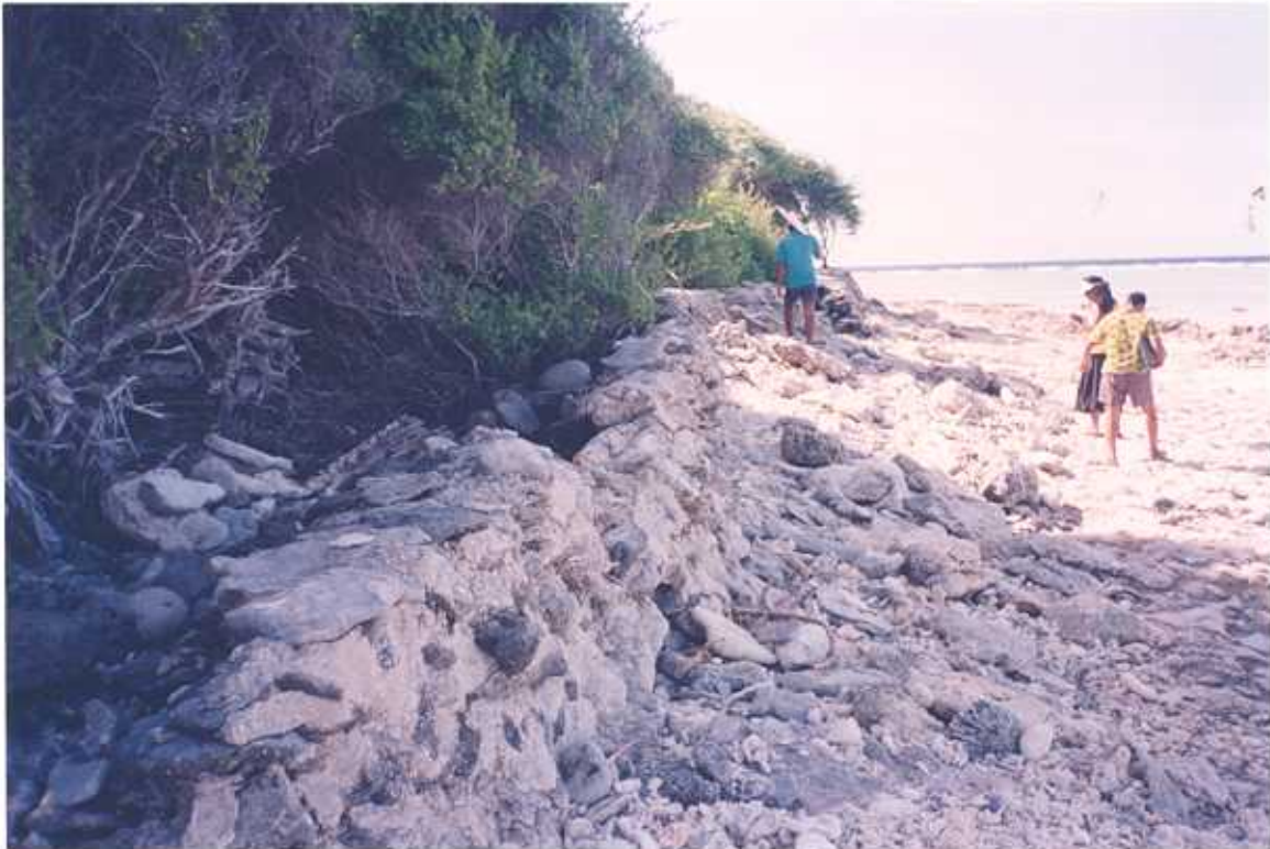
Figure 47. Taubukintekira (east of airfield), Kuria. View northwest near "east point" showing cemented coral rubble seawall. Seawall rests on a foundation of coral rubble overlying conglomerate platform.
