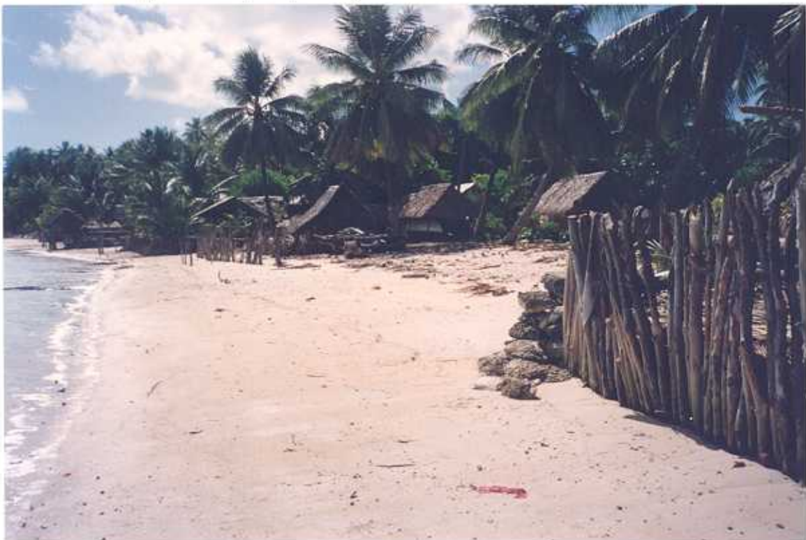
Figure 13. Maneaba at Nikutoru, Tabiteuea South. View northwest along lagoon shoreline beach illustrating local foreshore protection and/or land reclamation methods and the proximity of buildings to the shoreline.
