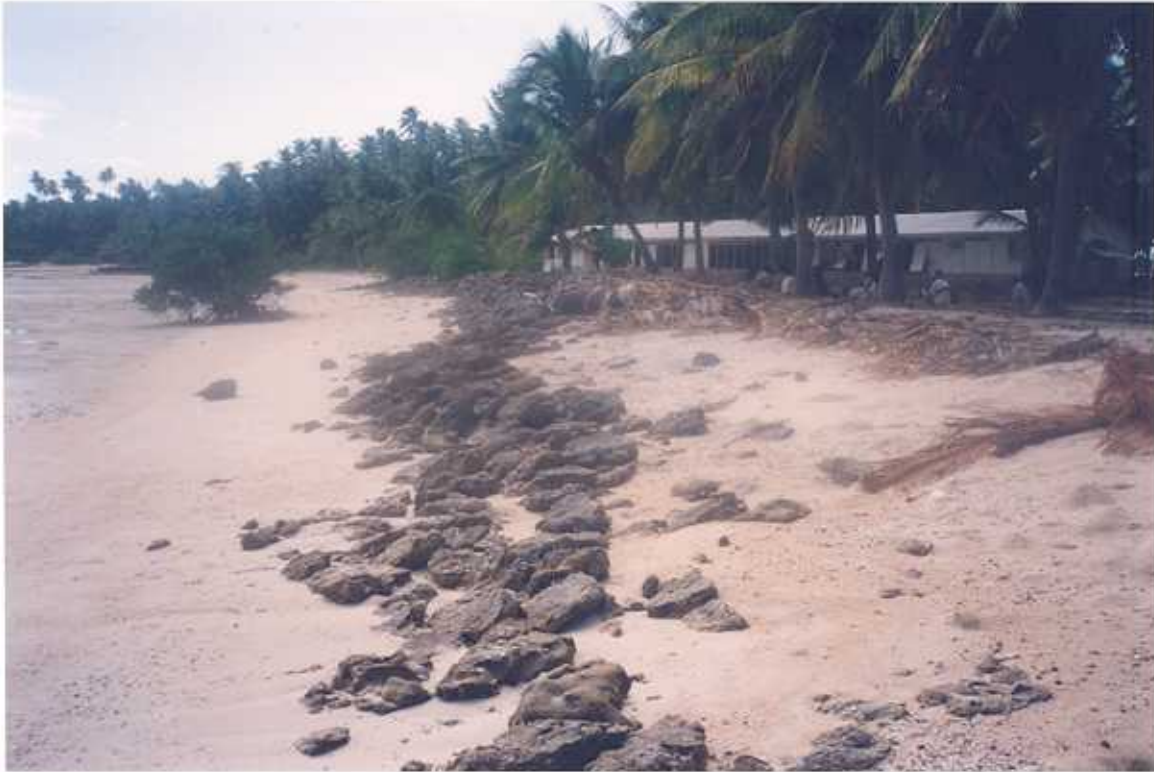
Figure 16. School at Tewai, Tabiteuea South. View northeast along lagoon/channel shoreline showing location of erosion and remains of rubble seawall in front of school. According to local island sources erosion has amounted to about 30 m.
