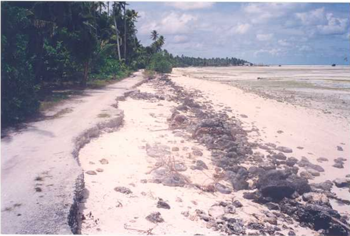
Figure 42. Tanimainiku (Beach Profile: 2), Abemama. View southeast past location of beach profile. Note severe erosion of road and remains of coral rubble seawall on beach.
