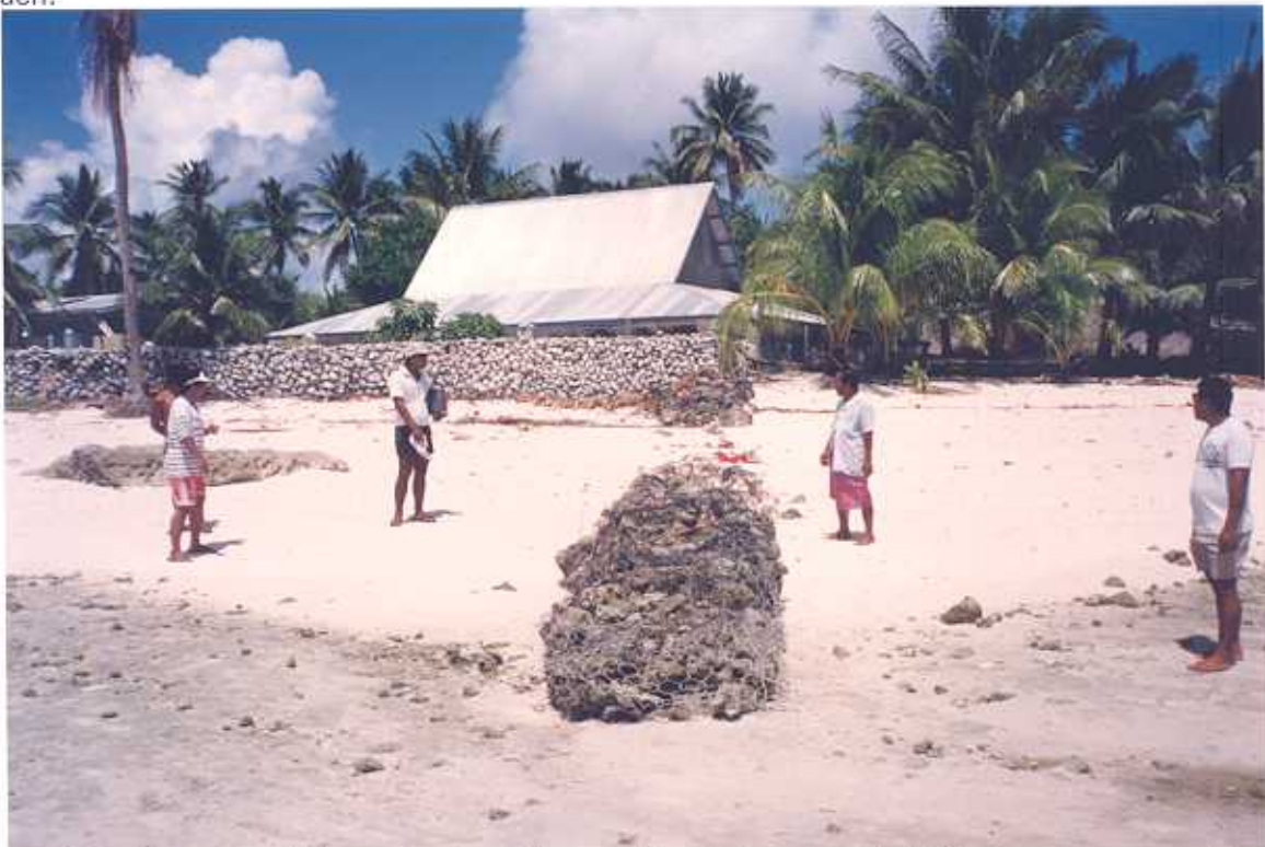
Figure 20. Tabuarorae Village, Onotoa. View southeast from reef flat. Photo shows seawall in front of maneaba and west of two gabion basket groynes. The beach profile runs down the beach to the right of gabion basket.
