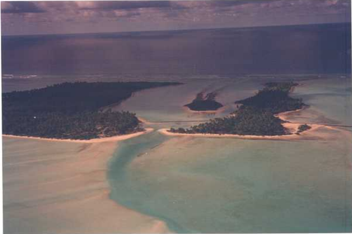
Figure 10. Aranuka Island, Tabiteuea South. View northeast to lagoon shoreline on Nikutiri Island (left) and Aranuka Island (right). Causeways joining islands have caused redistribution of lagoon shoreline sediments, specifically as erosion of island lagoon beaches and formation of lagoon spits across inter-islet channels. Note that the channel between Aranuka and Nikutiri is almost closed by spit growth.
