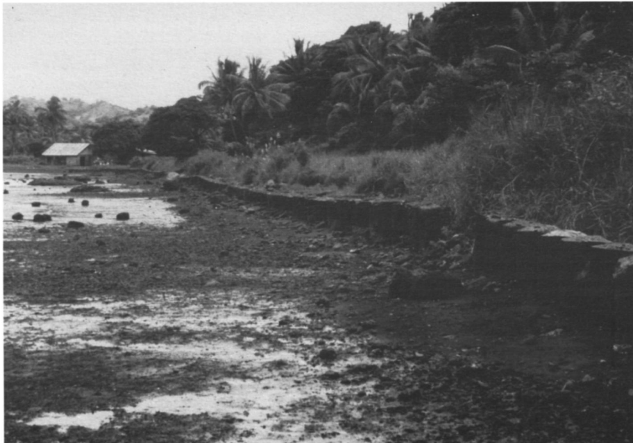
Plate 8. Vertical seawall of drums with concrete inside.
