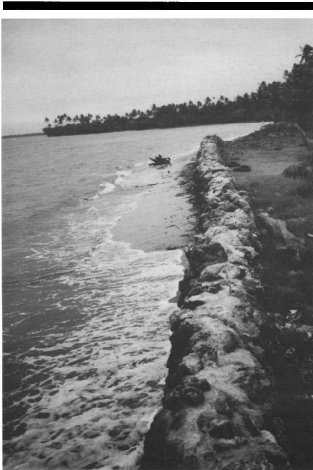
Plate 3. Seawall in front of Nukui village.
