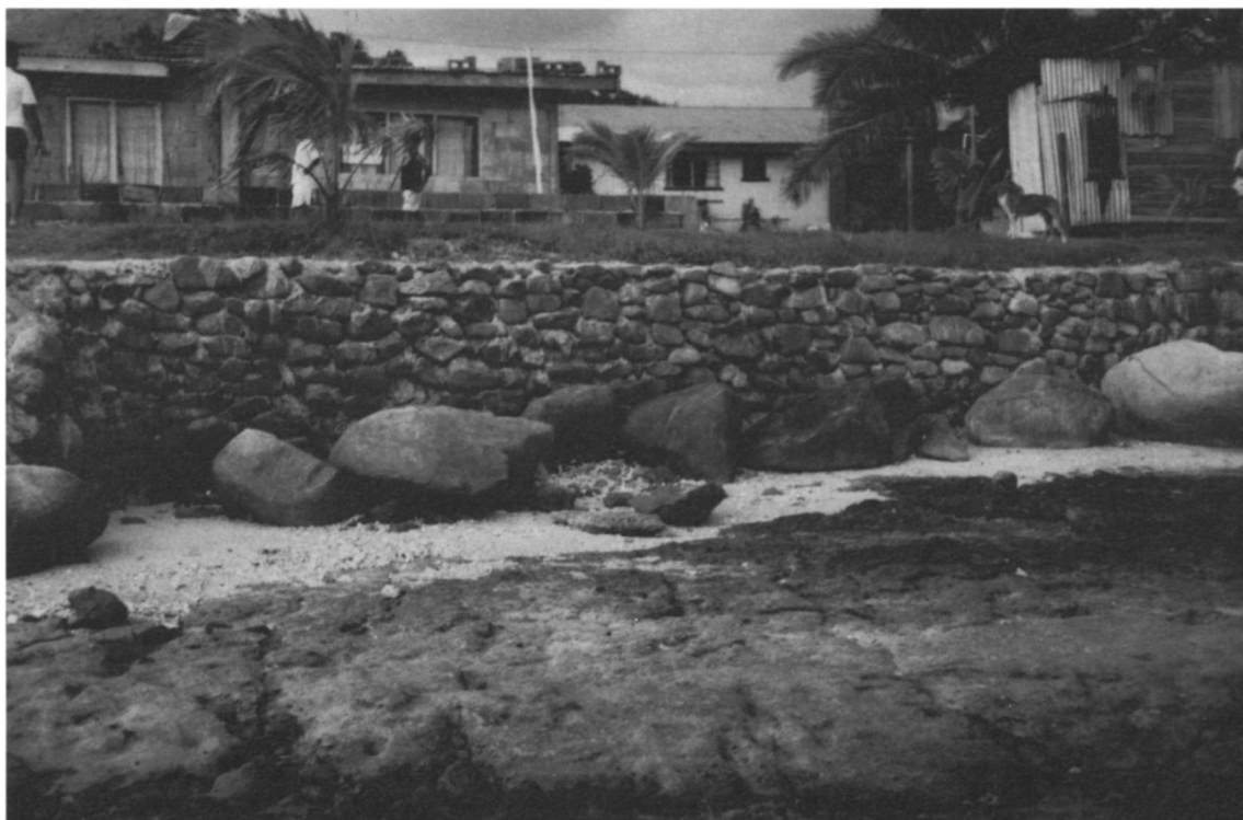
Plate 9. Vertical seawall with toe protection by large stones.
