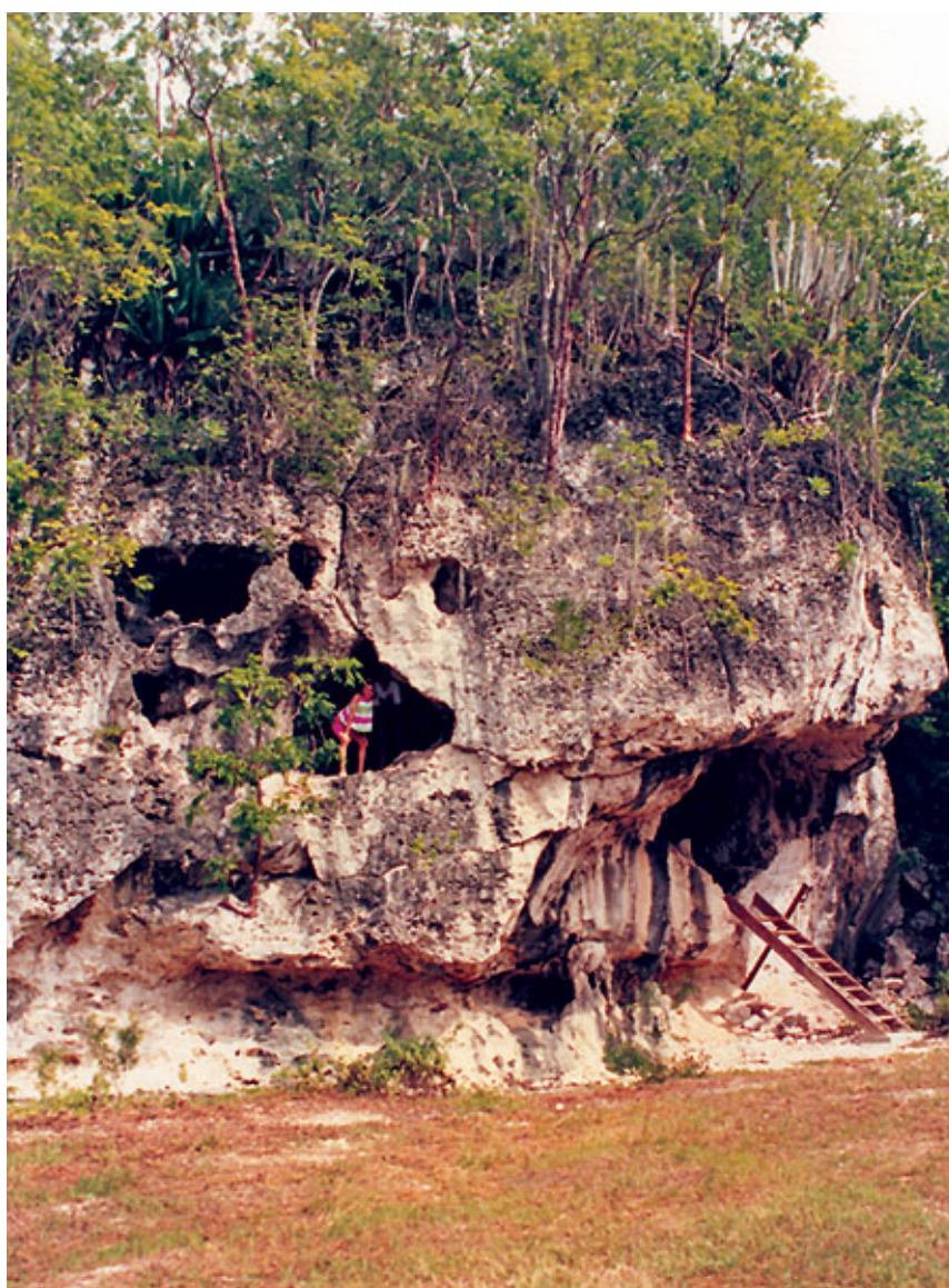
Figure 8. Erosion of the Bluff on Cayman Brac, Cayman Islands
