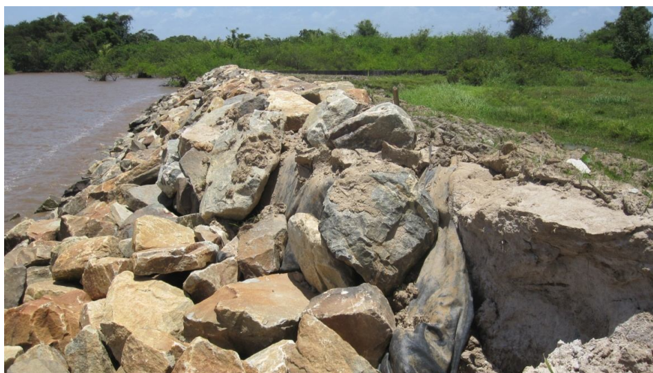
Figure 35: Guyana: Rehabilitation works completed at Henrietta
