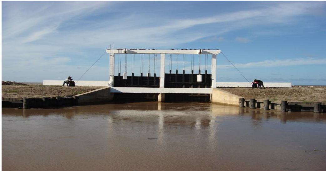
Figure 38: Drainage sluice
