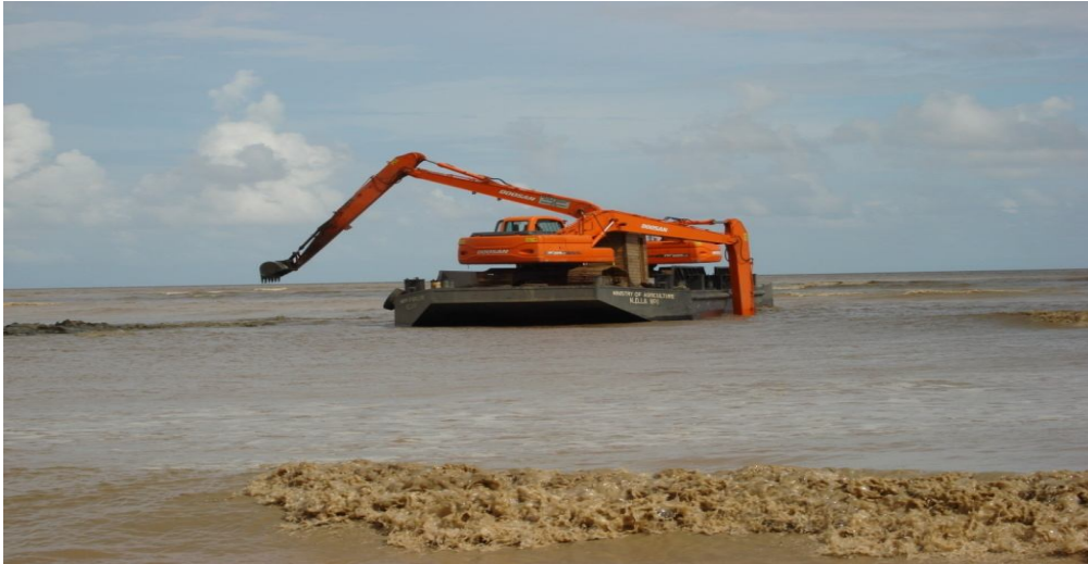
Figure 42: Dredging of sluices
