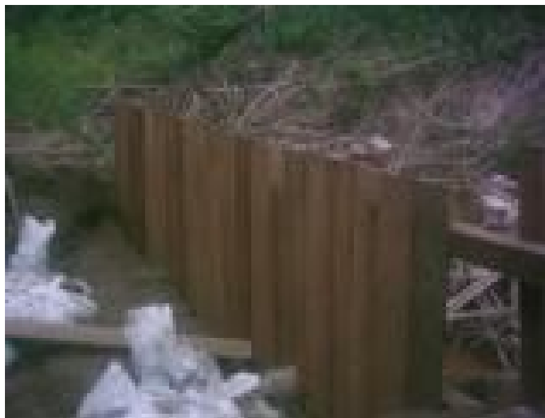
Figure 34: Revetment works at Friendship
