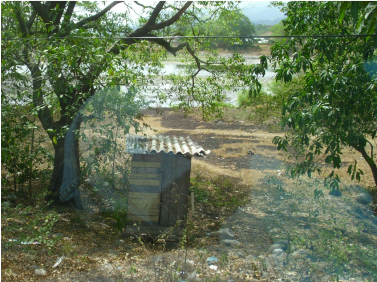
Figure 3-9: Household latrine in an informal settlement along the Cangrejal River
