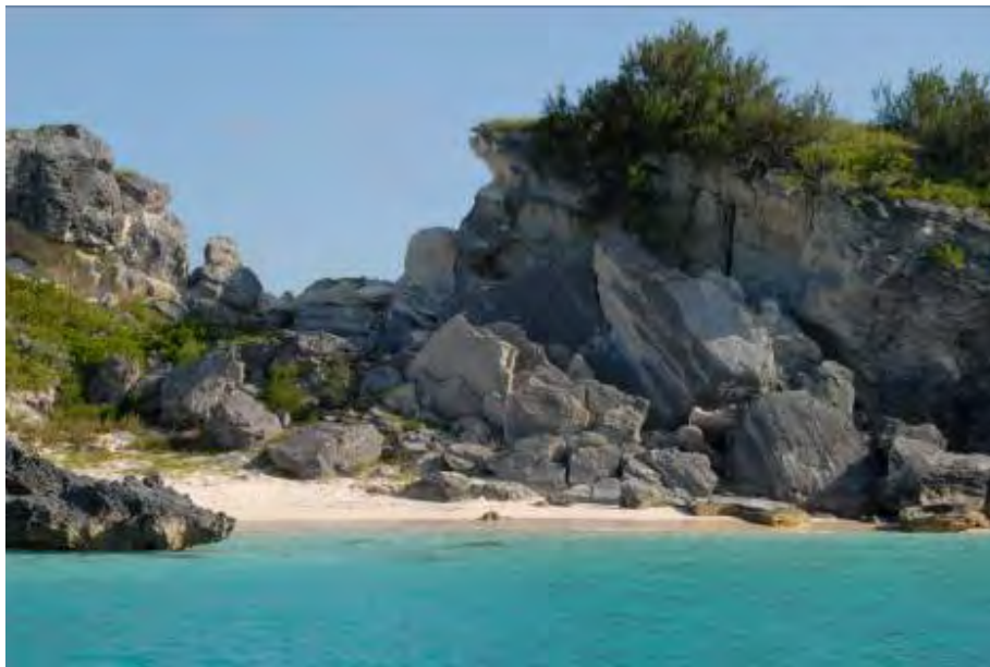
Photograph 9. Cliff collapse on Charles Island due to heavy rain.
