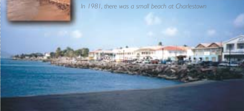
By 2000, the beach had disappeared and land has been reclaimed and protected with a boulder revetment
