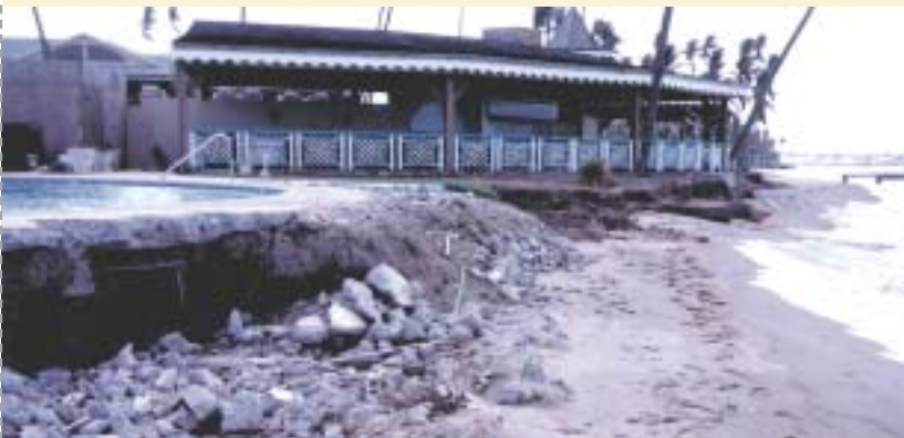
Pinney's Beach, October 1995, after Hurricane Luis
