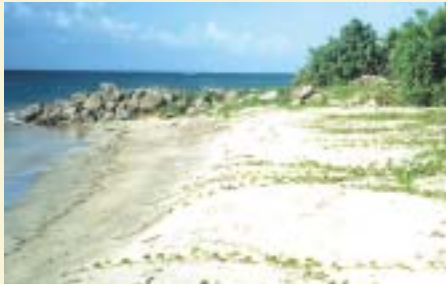
Groynes built along the north coast have stabilised the beach in some places (Newcastle 1997)...
