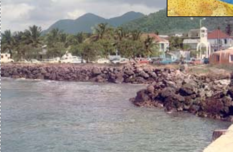
(below) Groynes, such as seen here at Sugar Bay in 1989, result in sand build-up on one side, but erosion on the other side
