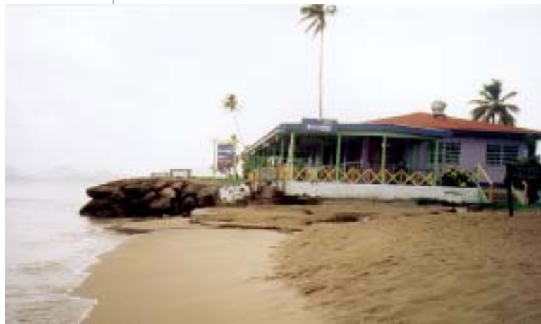
Armouring the shoreline, such as here at Pigeon Point, St Lucia, prevents access along the beach and causes conflicts 1997.
