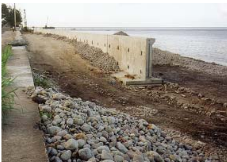
New seawall under construction, Ptitersville, Dominica 2001.
