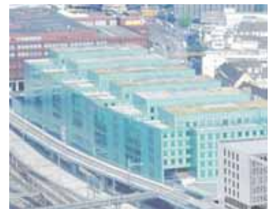
Figure 28: Green roofs on Peter Merian-Building in Basel. (Source: Zwimpfer Partner Architects.)
