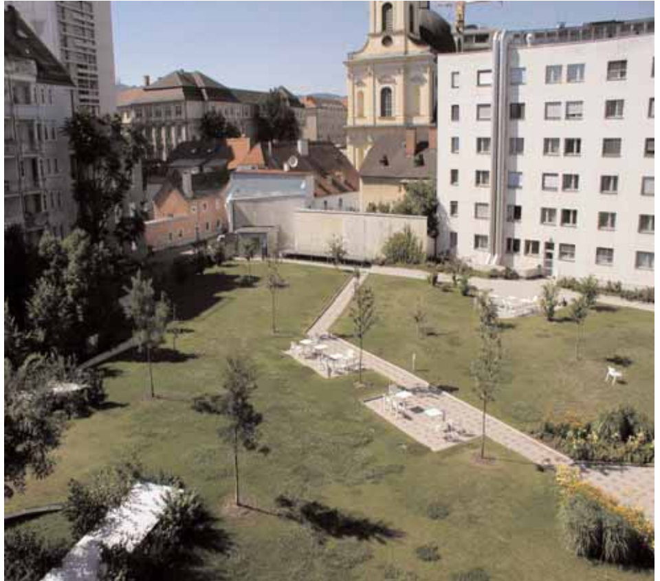
Figure 33: Green roof on a 2-storey underground garage. (Source: Municipal Planning board of Linz, Austria.)
