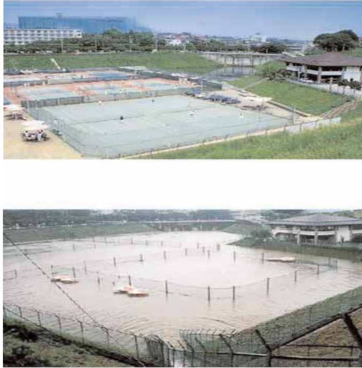
Figure 21: Yokohama rainwater detention reservoir under normal (dry) conditions (above) and flooded after a period of heavy rainfall (below). (Source: Ikeda, T. 2005, as above.)
