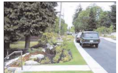
Figure 25: Narrow streets, bordered by beds of dense planting, minimise runoff and promote natural infiltration in the Broadview Green Grid neighbourhood. (Source: © 2005, Seattle Public Utilities, City of Seattle, WA)
