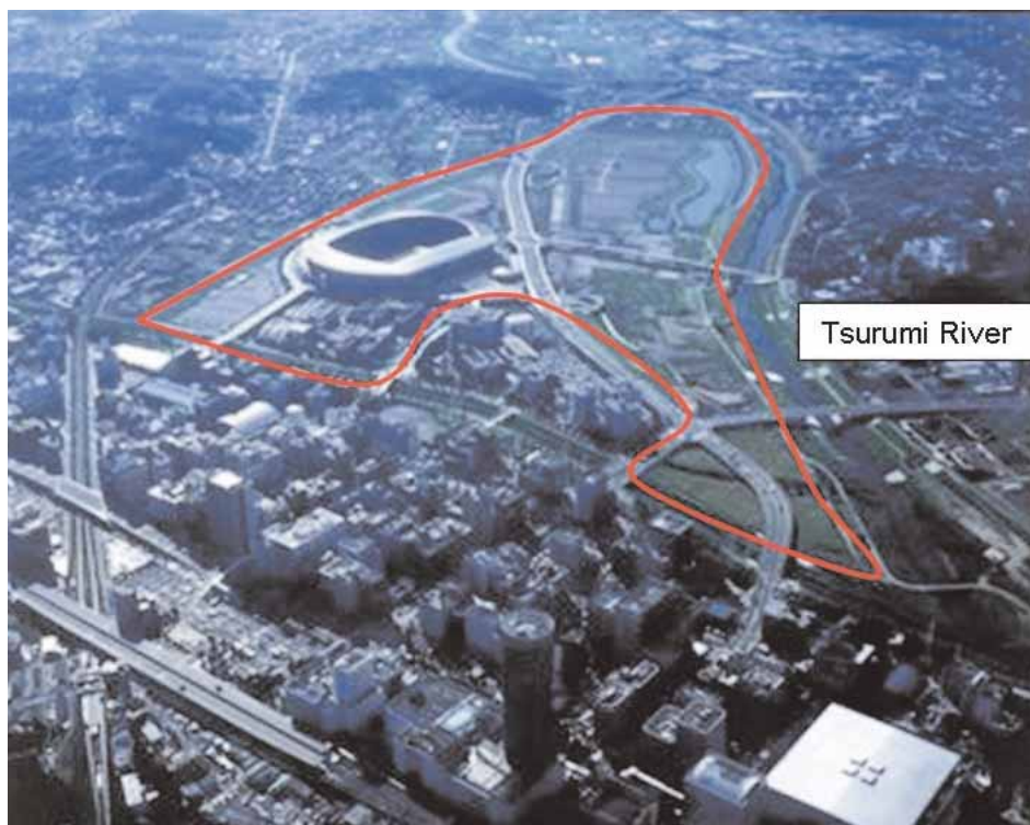
Figure 19: The Tsurumi River multipurpose retarding basin, with the International Stadium Yokohama as its centerpiece. (Source: Keihin Office of River Kanto Regional Development Bureau 19 )
