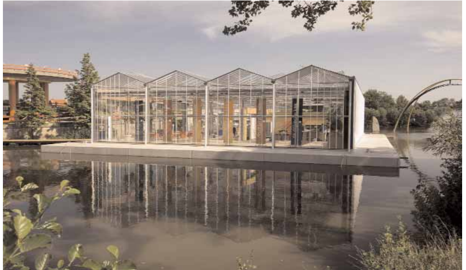
Figure 13: The Netherlands' first floating greenhouse. (Source: Dura Vermeer Groep NV.)
