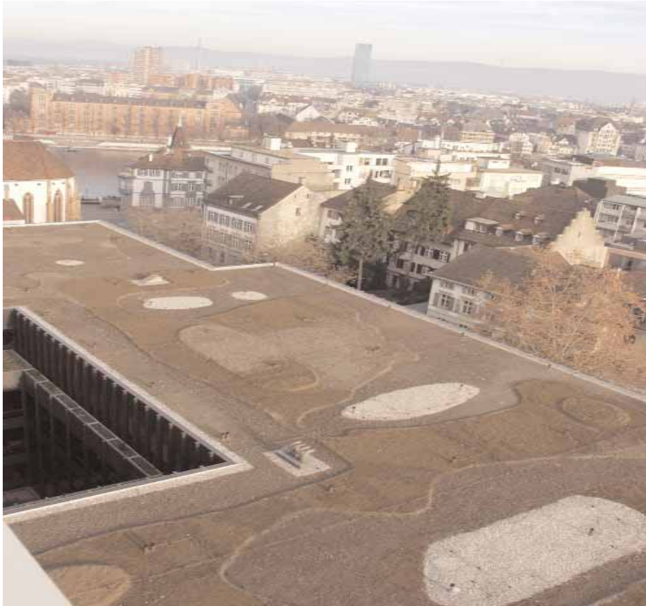
Figure 30: Newly constructed green roof on 'Klinikum 2' of Basel University Hospital, following the new guidelines in Basel's green roofs and urban biodiversity strategy (see Box). (Source: Stephan Brenneisen).
