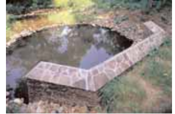
Figure 4: A typical outlet stilling basin in Staten Island's Bluebelt (Source: New York City Department of Environmental Protection)
