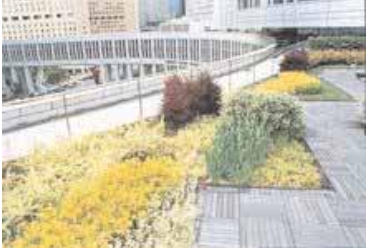
Figure 46: Green roof on the Tokyo Metropolitan Assembly Building. (Source: Tokyo Metropolitan Government Bureau of Environment and Bureau of Urban Development.)
