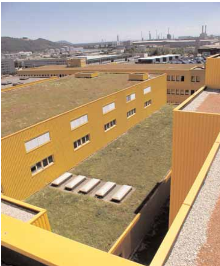
Figure 34: The Schachermayer factory has the largest area (more than 14,000 m 2 ) of extensive green roof in Linz and was the first to establish a self-funded green roof. (Source: Municipal Planning board of Linz, Austria.)
