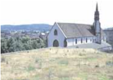
Figure 27: The green roof on Basel's University Hospital, which has been in place since the mid-1980s. (Source: Pia Zanetti).
