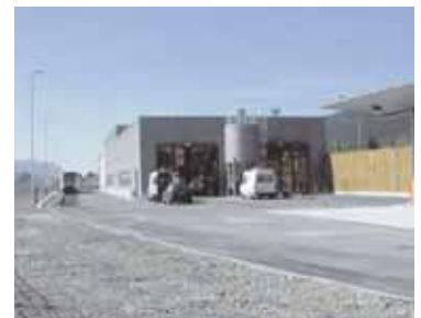
Figure 58: Internal and external views of the train maintenance depot owned by Hohenzollerische Landesbahn (HLZ), Germany (Source: Aquality Trading and Consulting Ltd.)
