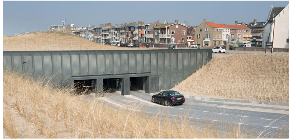
Multifunctional solutions for adapting coastal defenses: combining functions on top of and near coastal defenses creating added value in densely populated areas.
