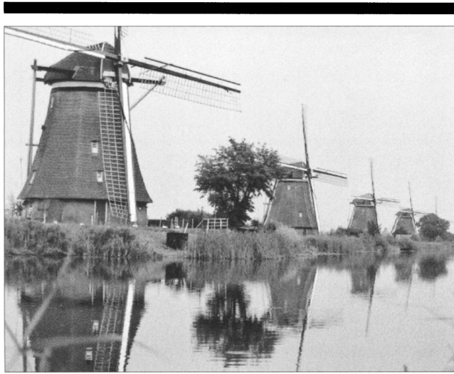
Figure 5. Drainage in stages by series of windmills (Courtesy of Rijkswaterstaat). For a color version of this figure, see page 445.
