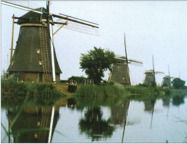
Figure 5. from “Living with Sea-Level Rise and Climate Change: A Case Study of the Netherlands” by M. VanKoningsveld, J.P.M. Mulder, M.J.F. Stive, L. VanDerValk, and A.W. VanDerWeck, pp. 367–379. Drainage in stages by series of windmills (Rijkswaterstaat).
