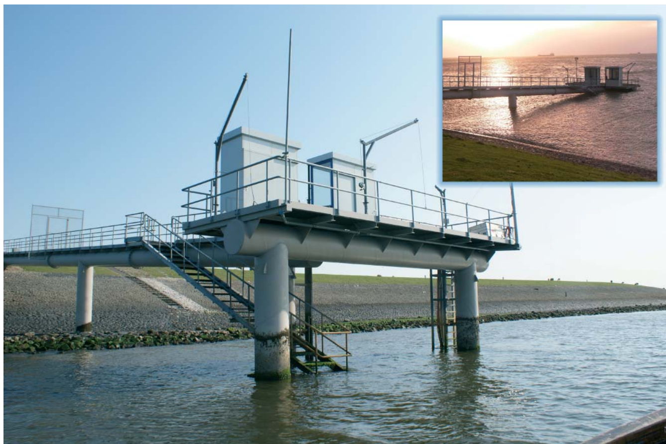
NIOZ is running a long-term measurement series of physical, chemical and biological measurements in the Marsdiep tidal inlet of the Western Wadden Sea from its own jetty. In 2007 an entirely new jetty was built; with a platform which has been elevated 2.7 m above the level of the old jetty. This proved to be high enough to withstand the extremely high-tide at 9 November 2007. Photos: Jan Boon (NIOZ).
