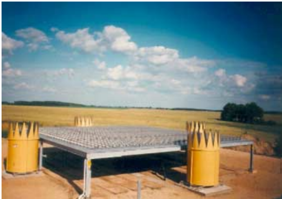
Fig. VIII.6.6.1 "LAP – 16000" tropospheric wind profiler / RASS at the Lindenberg Meteorological Observatory (German Weather Service)
