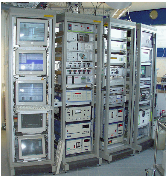
Fig. VIII.6.4.1 GAW – Schauinsland regional station of the Federal Environmental Agency
