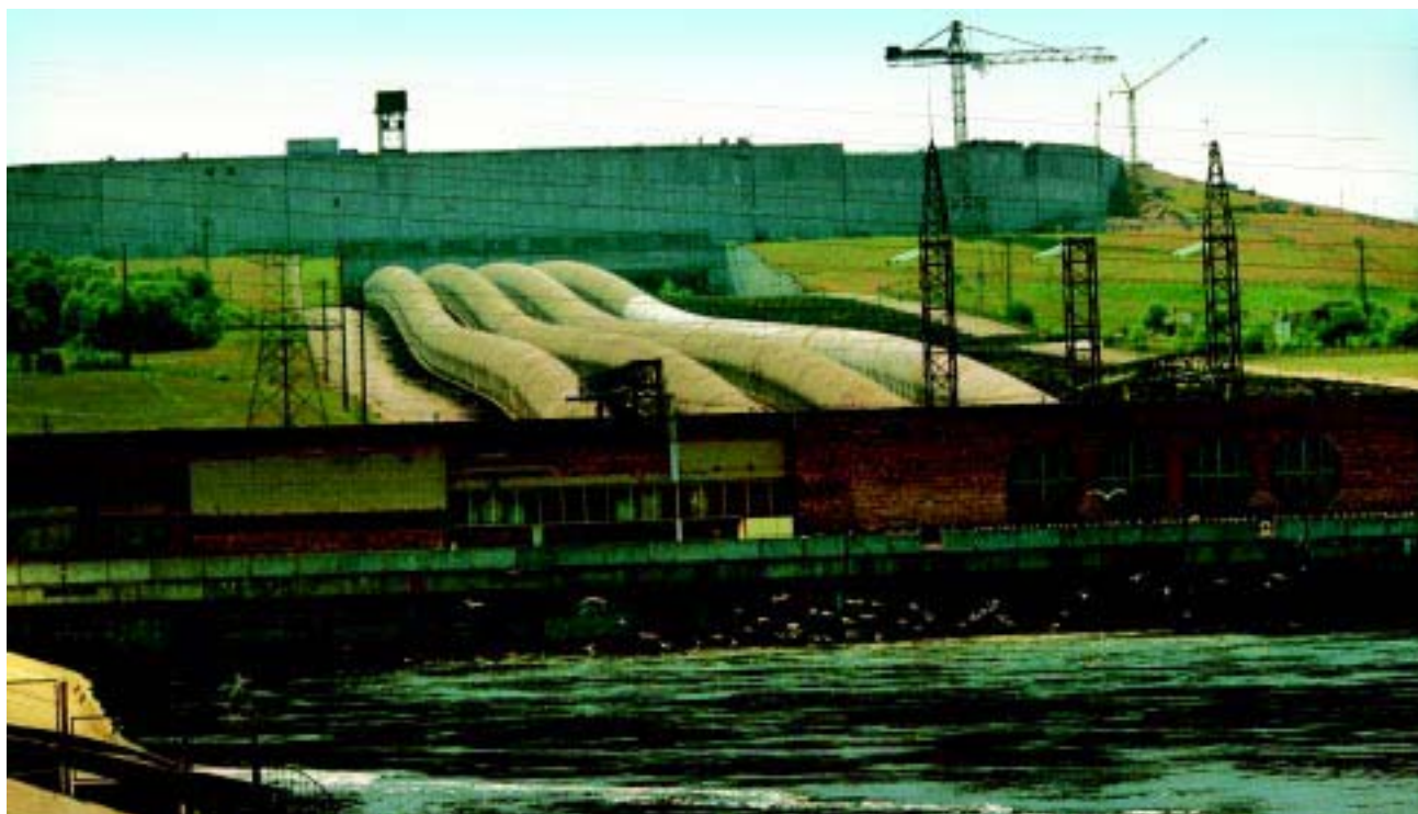
Kruonis Hidro-Accumulation plant
