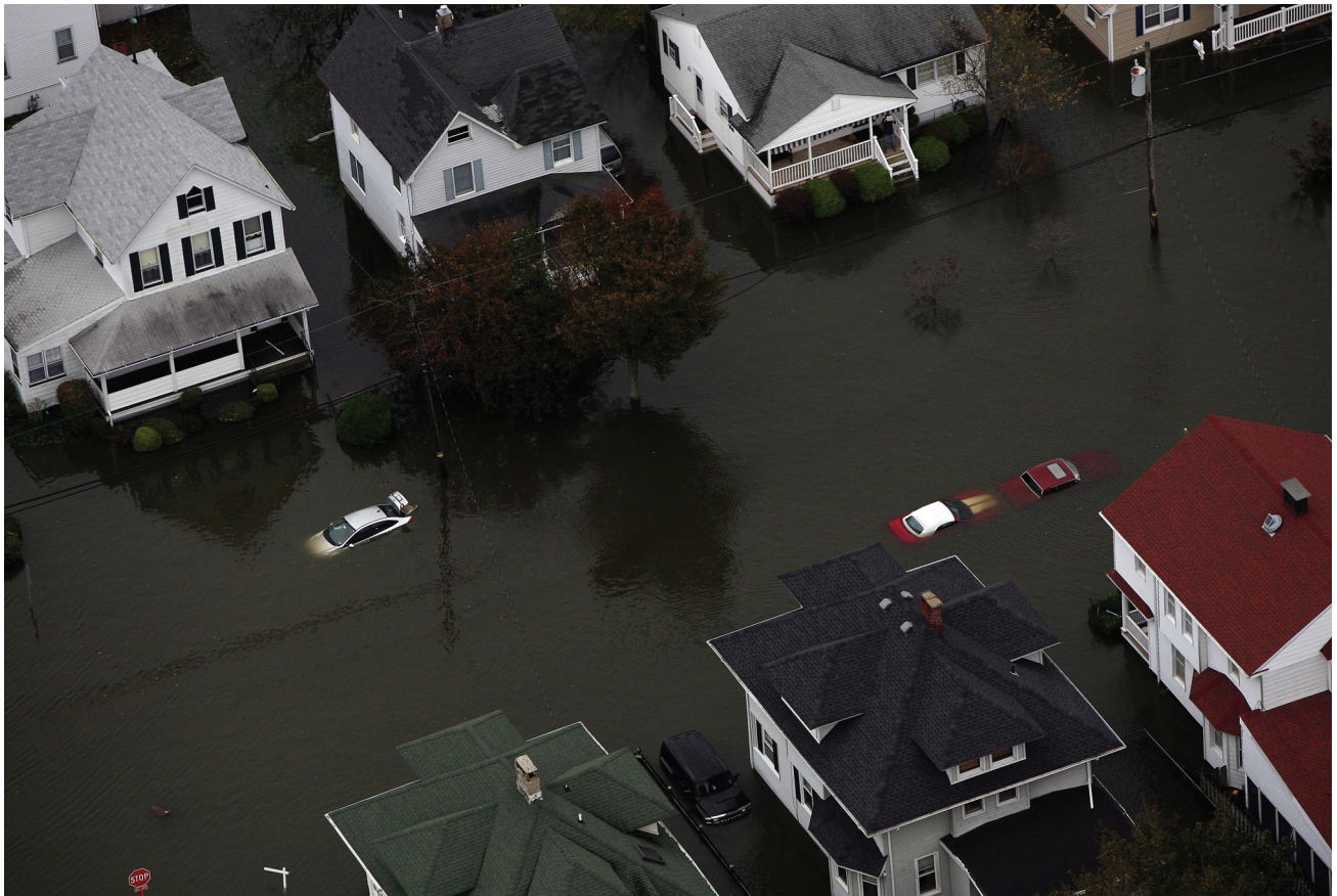
Figure 10: Hurricane Sandy damage in Belmar, N.J. on Tuesday, October 30, 2012
