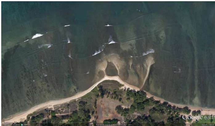
GROYNE-LIKE STRUCTURES IN KIHEI, MAUI, HI. (IMAGE SOURCE: GOOGLE EARTH 2 )
