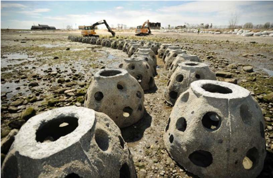
REEF BALL INSTALLATION. (IMAGE SOURCE: BRIAN A. POUNDS, CONNECTICUT POST 7 )
