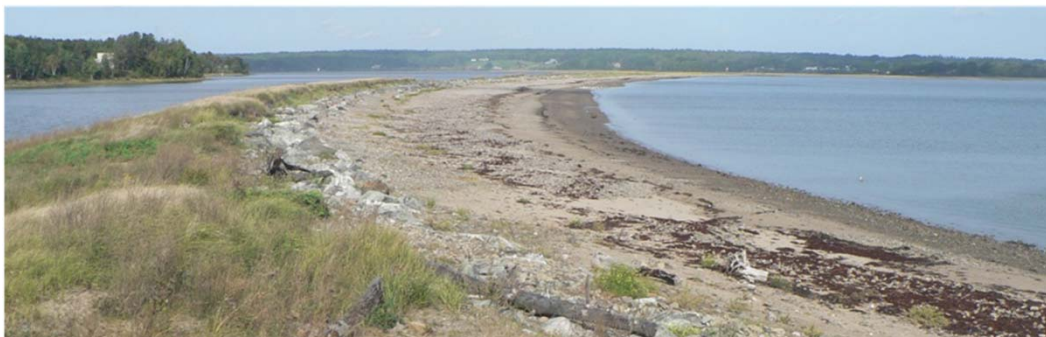
BURIED REVETMENTS AT DOMINION BEACH, NS, TWO YEARS AFTER CONSTRUCTION (TOP), AND LIGHTHOUSE BEACH, NS, SIX YEARS AFTER CONSTRUCTION. (IMAGE SOURCES: VINCENT LEYS, CBCL LIMITED)
