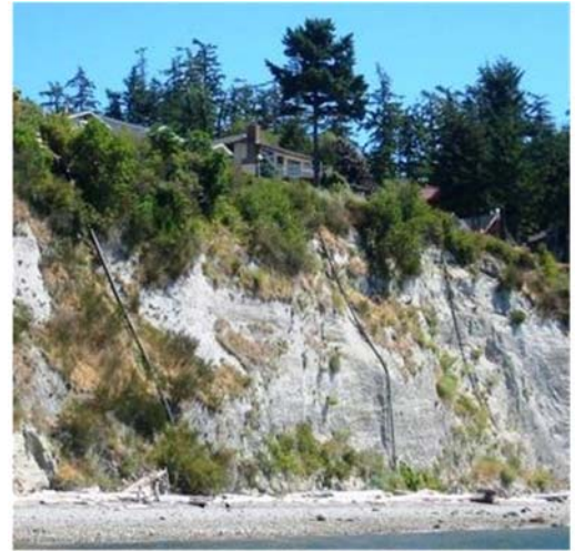
EXAMPLE OF TIGHTLINE DRAINAGE IN WASHINGTON. (IMAGE SOURCE: STATE OF WASHINGTON DEPARTMENT OF ECOLOGY 1 )
