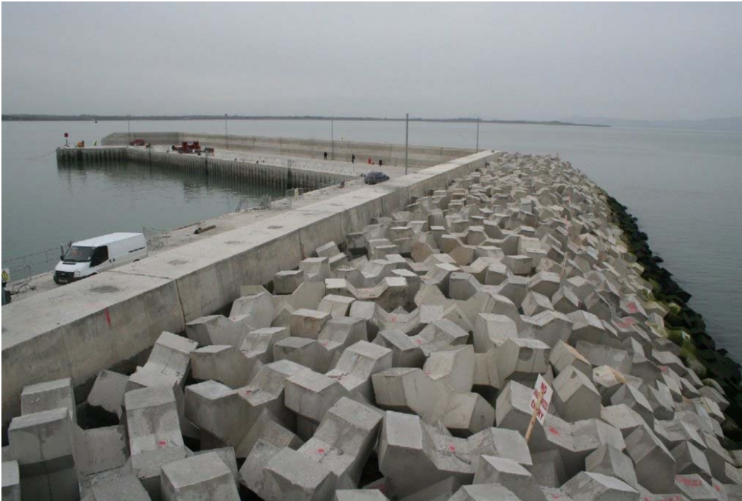
COMPLETED BREAKWATER WITH XBLOC ARMOUR LAYER AT PORT ORIEL. (IMAGE SOURCE: XBLOC 1 )
