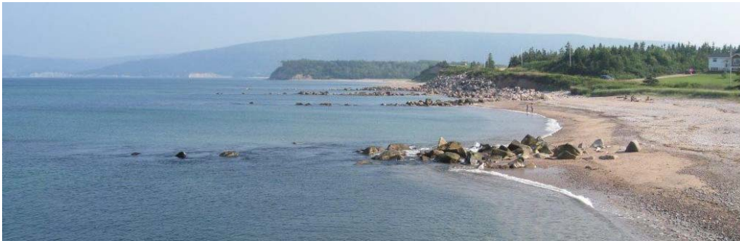
LOW-CRESTED GROYNES AT DINGWALL, NS. (IMAGE SOURCE: VINCENT LEYS, CBCL LIMITED)
