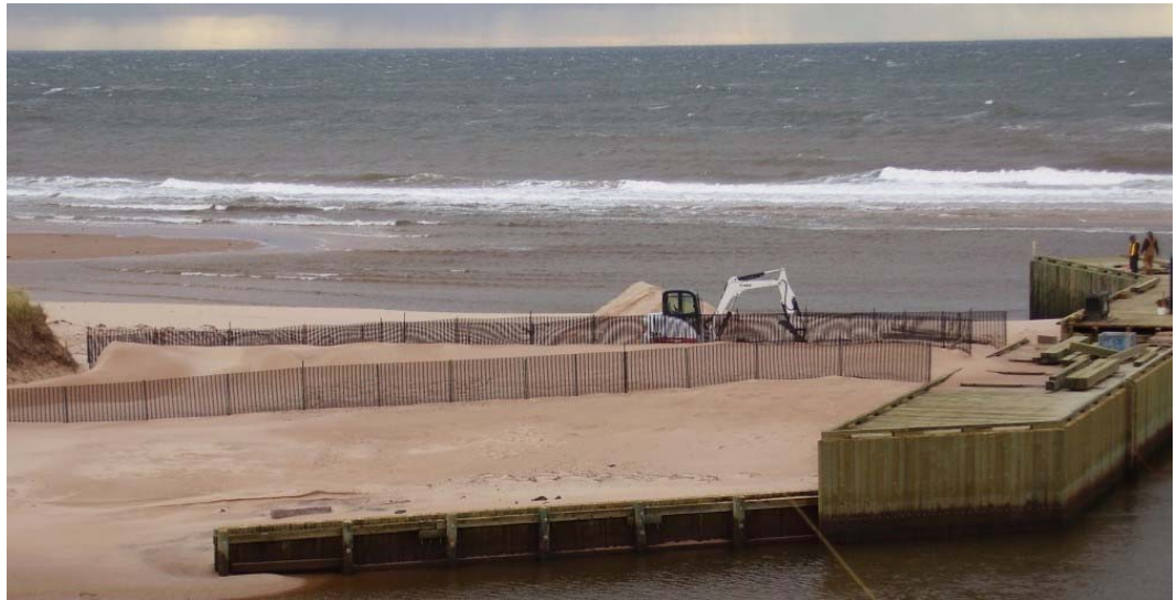
DUNE RESTORATION DURING THE CONSTRUCTION OF A BURIED REVETMENT AT BASIN HEAD, PEI. (IMAGE SOURCE: JODY MACLEOD, CBCL LIMITED)
