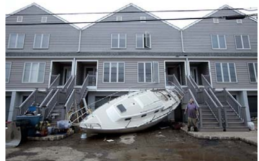
IMPACT ON THIS FLOOD-PROOFED HOUSING IS MINIMAL DESPITE MAJOR IMPACTS TO SEA BRIGHT SHORELINE INFRASTRUCTURE AS INDICATED BY THE BEACHED SAIL BOAT. (IMAGE SOURCE: STAR-LEDGER 6 )
