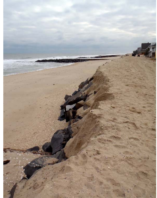
BURIED REVETMENT POST-HURRICANE SANDY. (IMAGE SOURCE: JENNIFER IRISH 3 )
