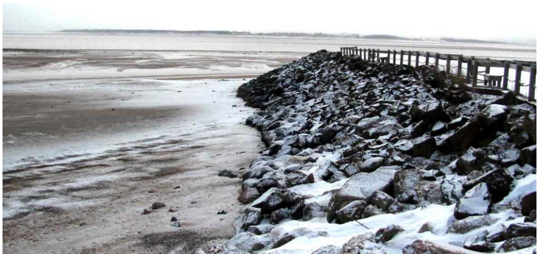
RIP-RAP SLOPE AT KINGSPORT, NS, ON THE BAY OF FUNDY. (IMAGE SOURCE: BRUCE HIGGINS, CBCL LIMITED)
