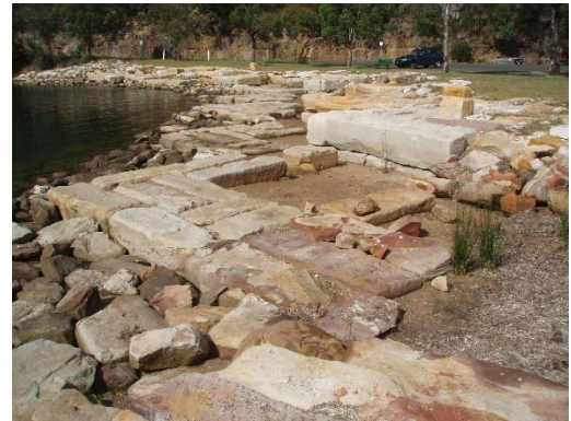
BOBBIN HEAD SEAWALL. (IMAGE SOURCE: D. WIECEK, OFFICE OF ENVIRONMENT AND HERITAGE)
