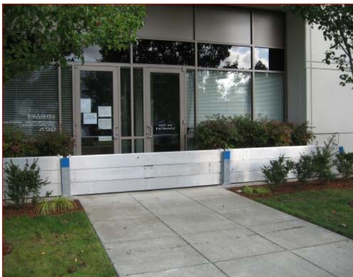
EXAMPLE OF A REMOVABLE FLOODWALL/GATE IN MAINE. (IMAGE SOURCE: FLOOD CONTROL AMERICA 9 )
