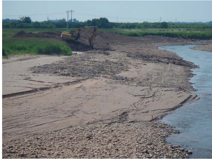
EXAMPLE OF A DREDGING PROJECT FROM A SMALL-SCALE CHANNEL MECHANICAL EXCAVATION IN SALMON RIVER, NOVA SCOTIA. (IMAGE SOURCE: GRAEME MATHESON, SAINT MARY'S UNIVERSITY)
