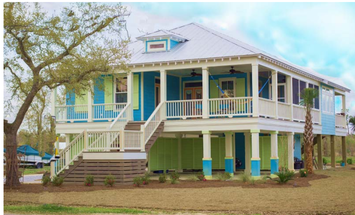
EXAMPLE OF A RAISED HOUSE IN WAVELAND, MISSISSIPPI. (IMAGE SOURCE: THORNHILL CONSTRUCTION 5 )
