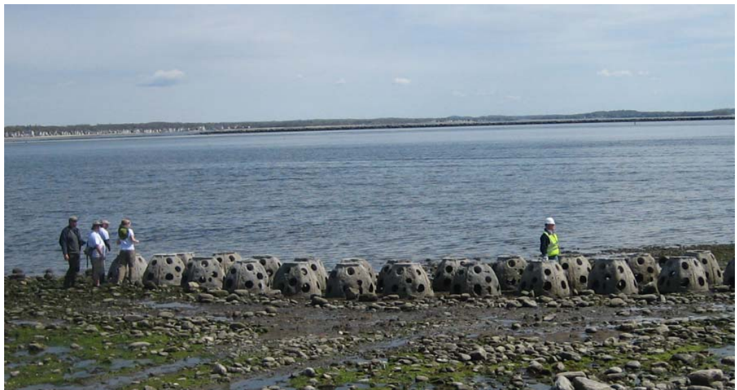
CONCRETE REEF BALLS. (IMAGE SOURCE: PAUL STERN, THE CT MIRROR 3 )
