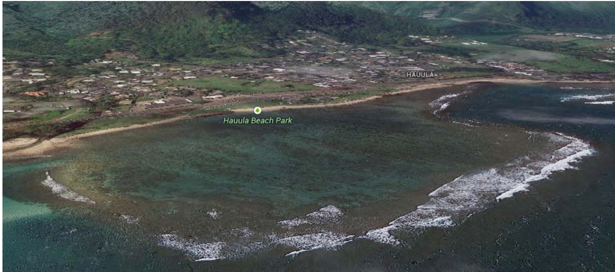
NATURAL REEF BREAKWATER AND GROYNES AT HAU'ULA, O'AHU. (IMAGE SOURCE: GOOGLE EARTH 3 )
