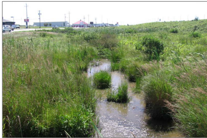
GRASS SWALE IN YARMOUTH, NOVA SCOTIA. (IMAGE SOURCE: ALEXANDER WILSON, CBCL LIMITED)
