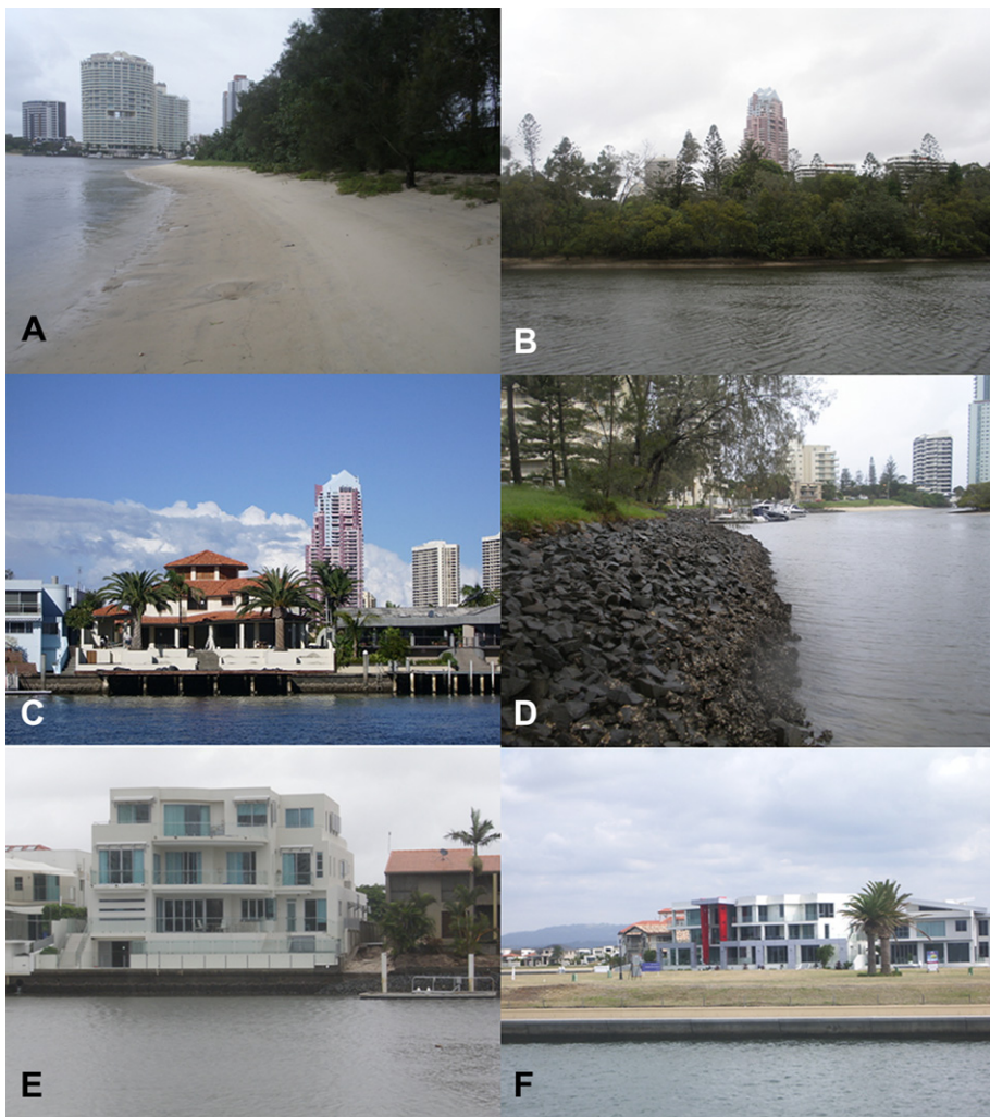
Fig. 7. Various forms of shoreline on the lagoon margins. A, B, Natural shorelines comprising sand and mangroves. C. Quays and revetments, D. Rock armour, E, F. Revetments.
