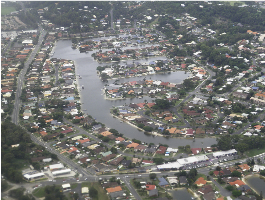
Fig. 6. Oblique aerial view of dense low-rise development around lagoon shoreline.
