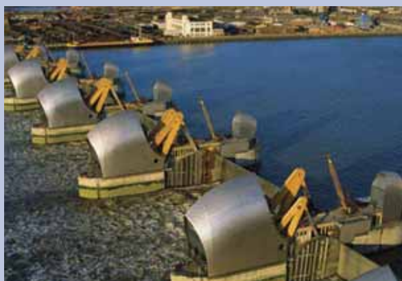
The retractable barrier on the Thames River, United Kingdom.
