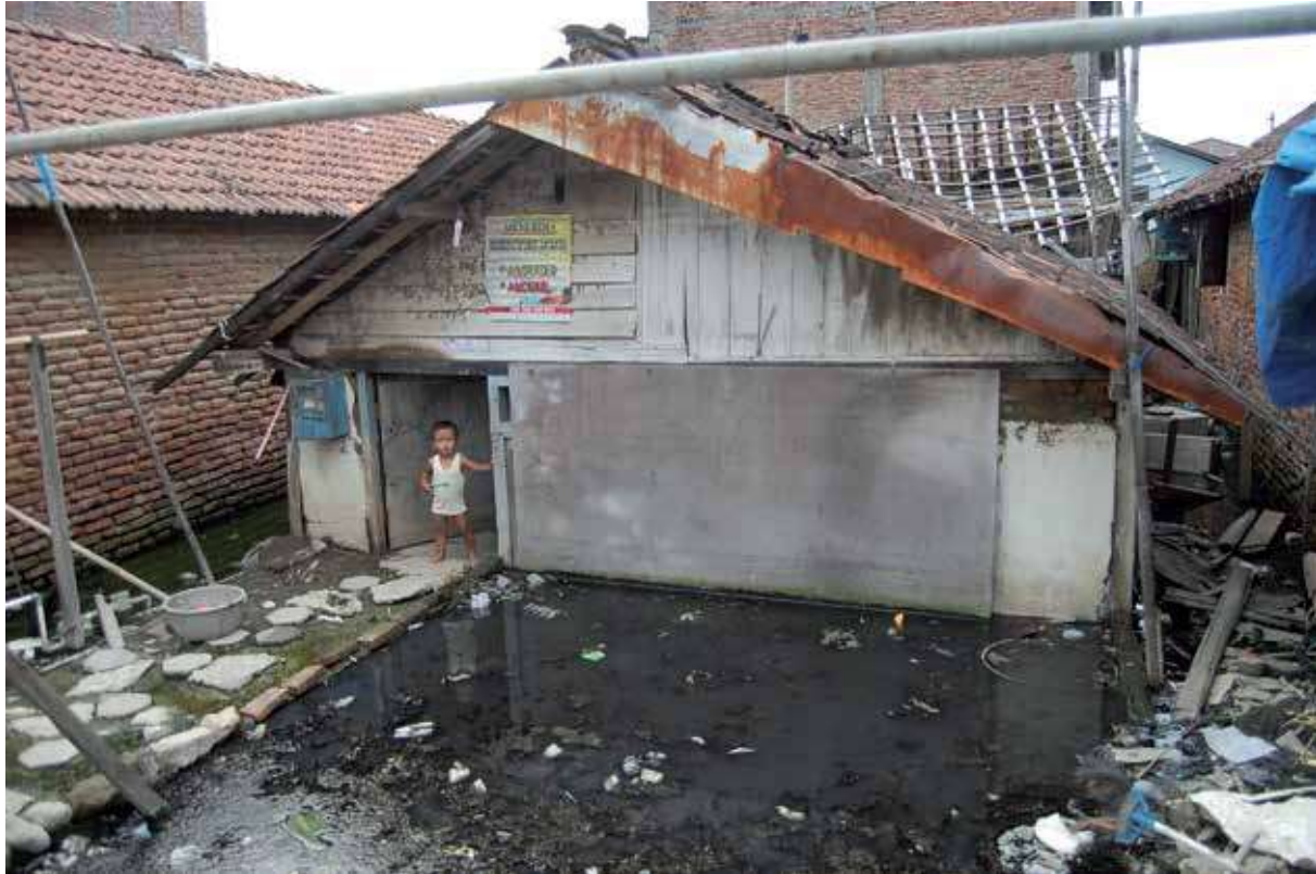
Figure 8. Vulnerable house in Tanjung Mas
