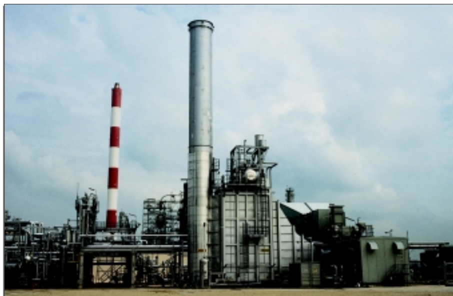
A co-generation plant of an oil refinery. (Picture courtesy of Shell Eastern Petroleum (Pte.) Ltd.)
