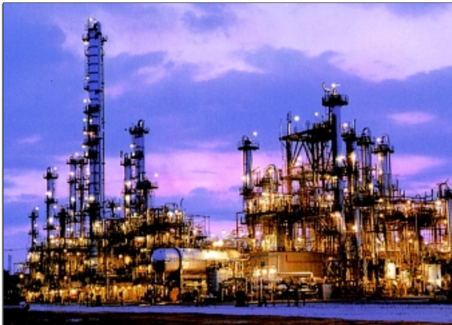
A petro-chemical plant. (Picture courtesy of Eastman Chemical Singapore Pte. Ltd.)
