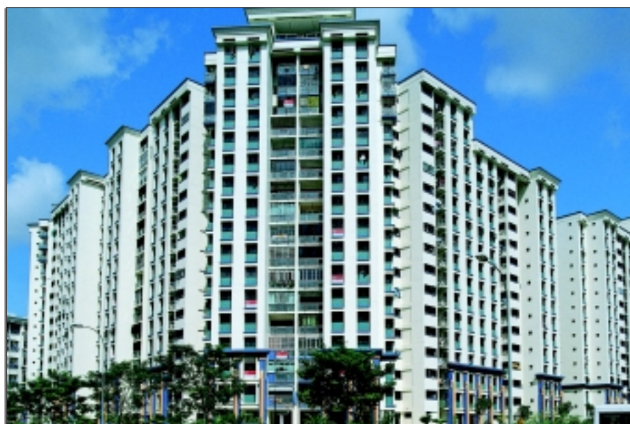
Public housing designed for optimal natural ventilation.
