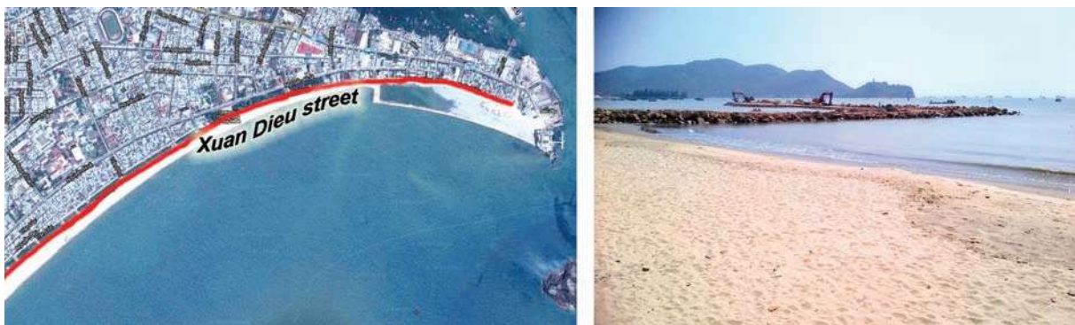
Figure 15. Xuan Dieu Street: satellite image and embankment construction
